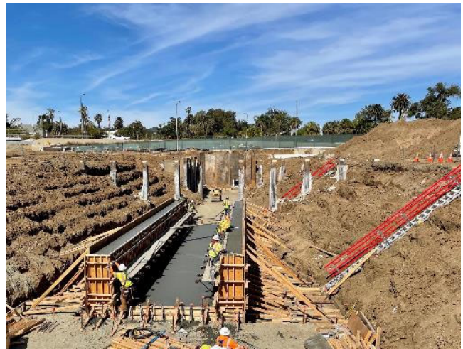
VA Steam Tunnel Relocation Concrete Pour for Reinforced Concrete Pipe Cradle
