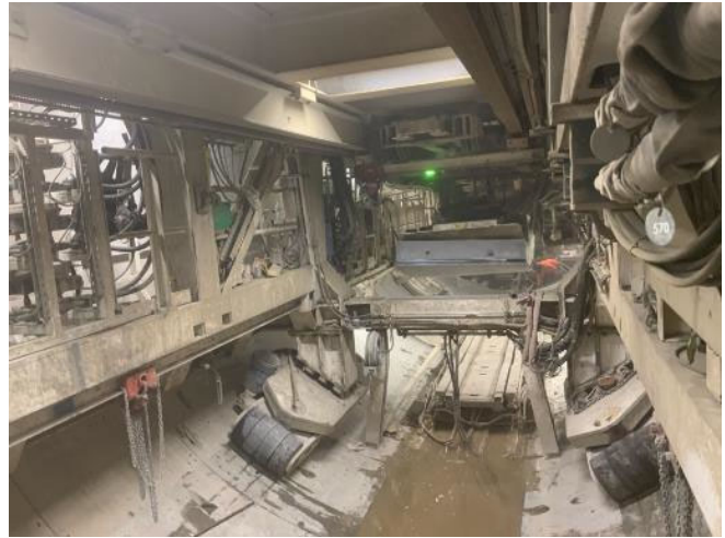
TBM Ring Segment Installation in BR Tunnel
