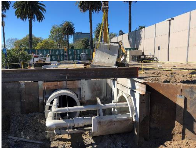
VA Steam Tunnel Vault 400 Sawcut and Remove Reinforced Concrete Pipe
