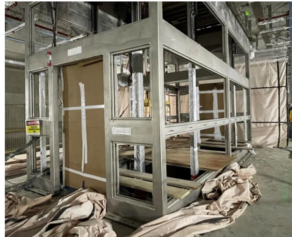
PL3/4 elevator at Platform Level for bead blasting at Historic Broadway Station
