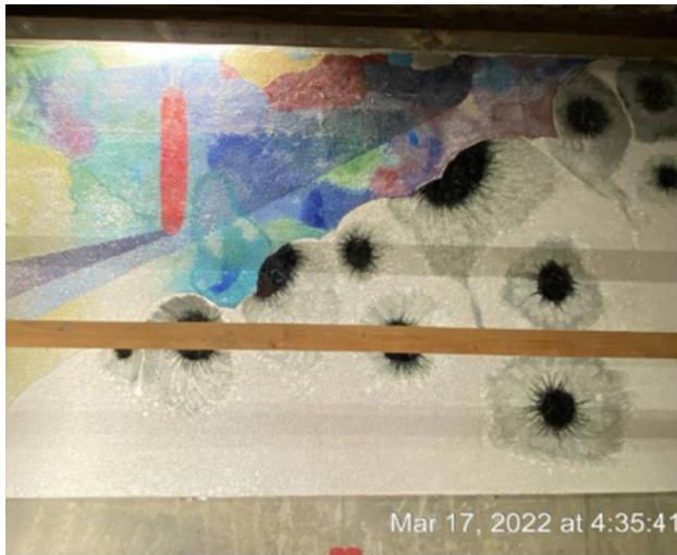
Mosaic Art Wall installation at Concourse Level
