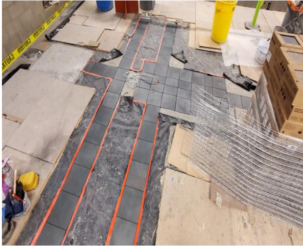
Ceramic tile installation at Platform Level
