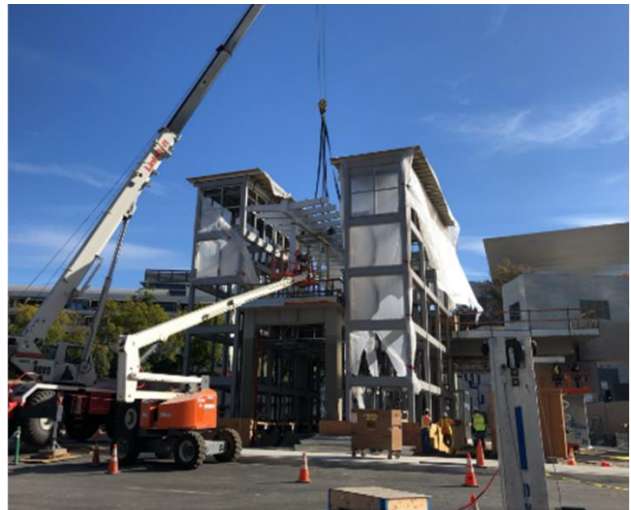
Plaza Level construction
