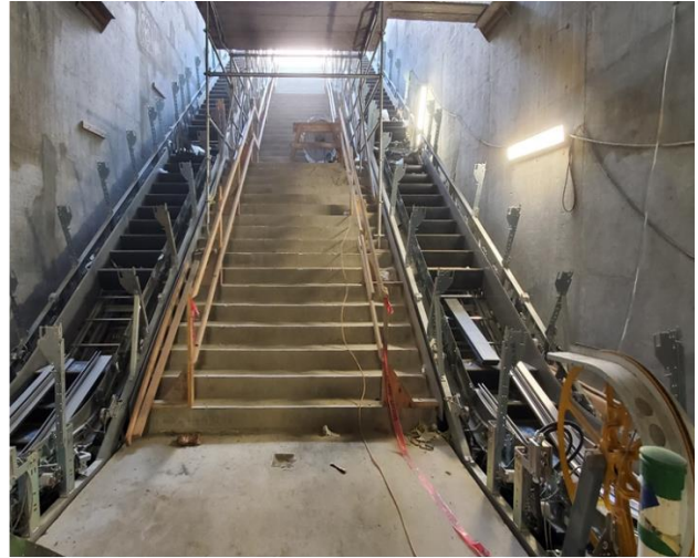
Installation of Public Escalators PE1 and PE2
