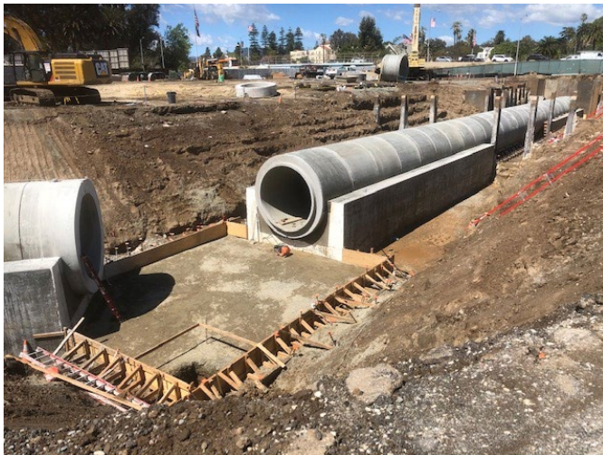
VA Steam Tunnel Reinforced Concrete Pipe Installation Between Vaults 300 and 200
