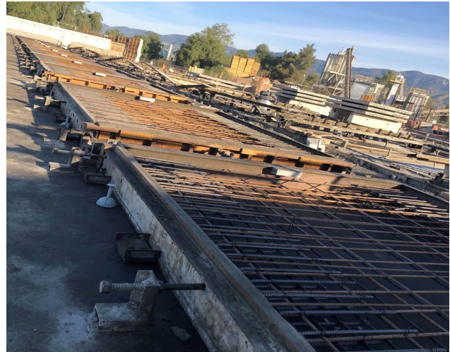
Westwood/UCLA Station Decking Panels Prepared Prior To Concrete Placement
