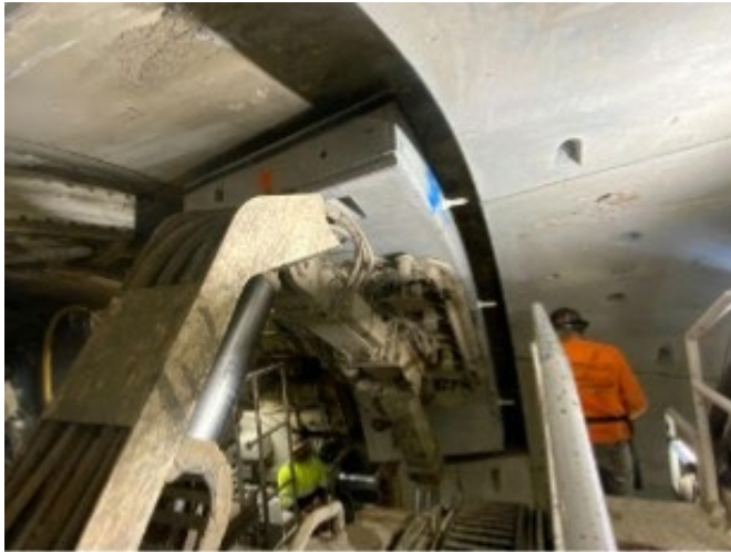
BL TBM Ring 803 Installation at UCLA Station
