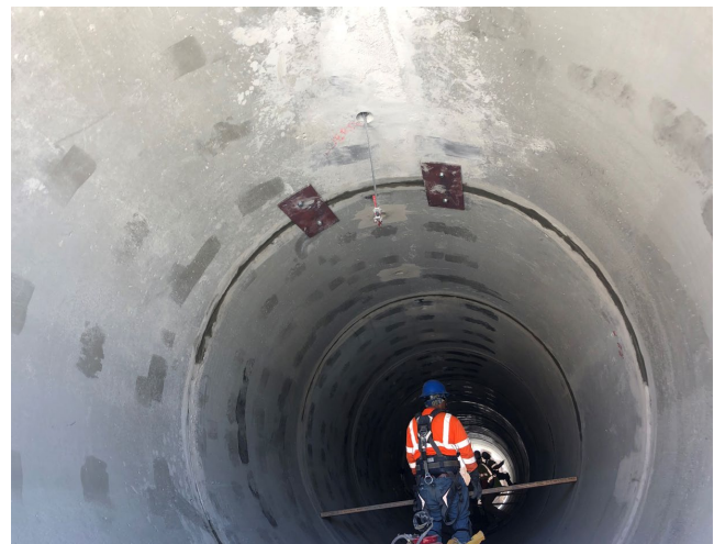
VA Steam Tunnel Finishing Works Within Reinforced Concrete Pipes
