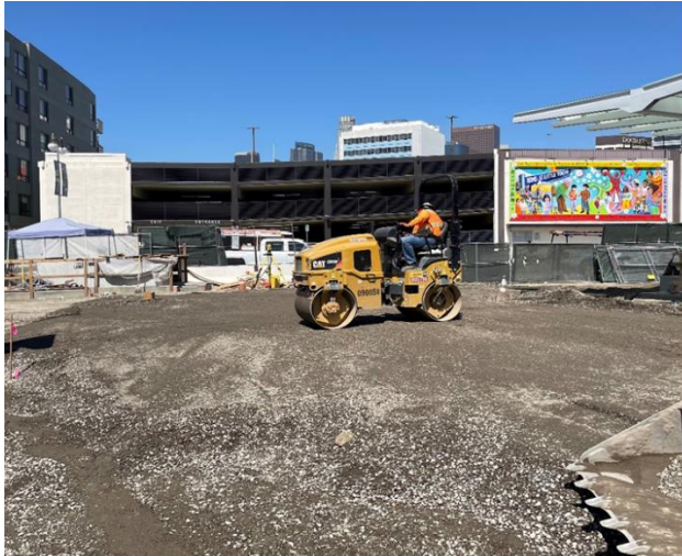
Plaza backfill progress at Little Tokyo/Arts District Station
