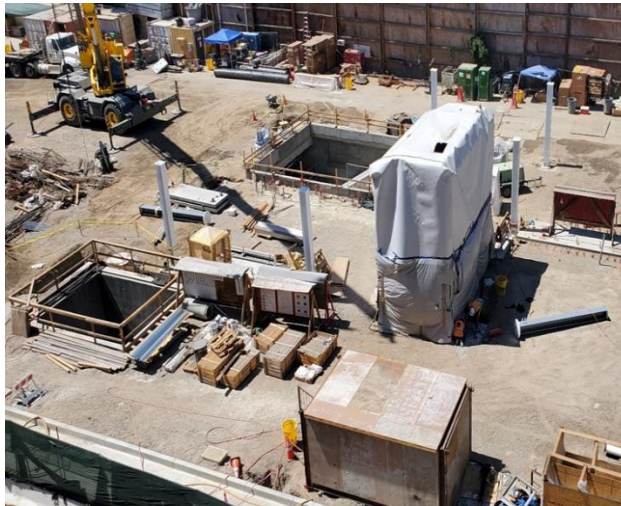
Canopy column construction at plaza level at Historic Broadway Station
