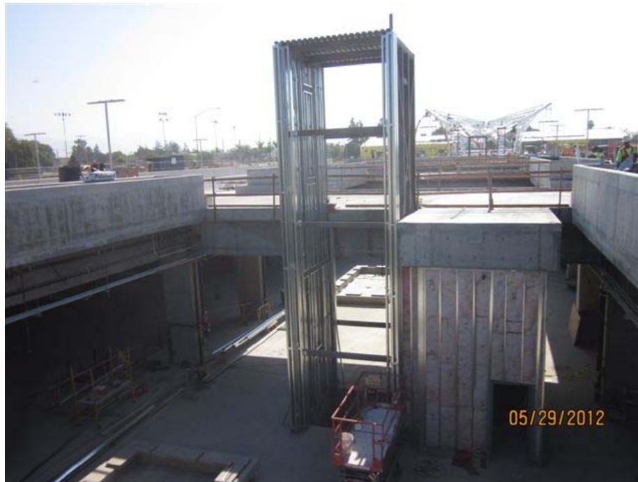
Metal framing on elevator shaft #3.
