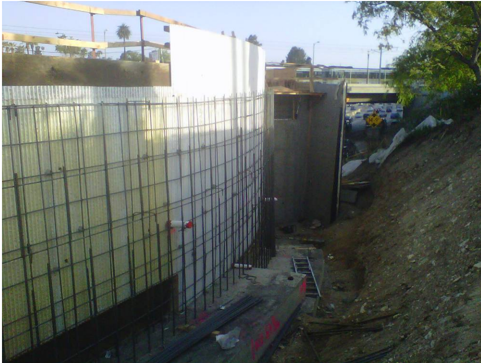
Area prepared for backfill behind POC wall.
