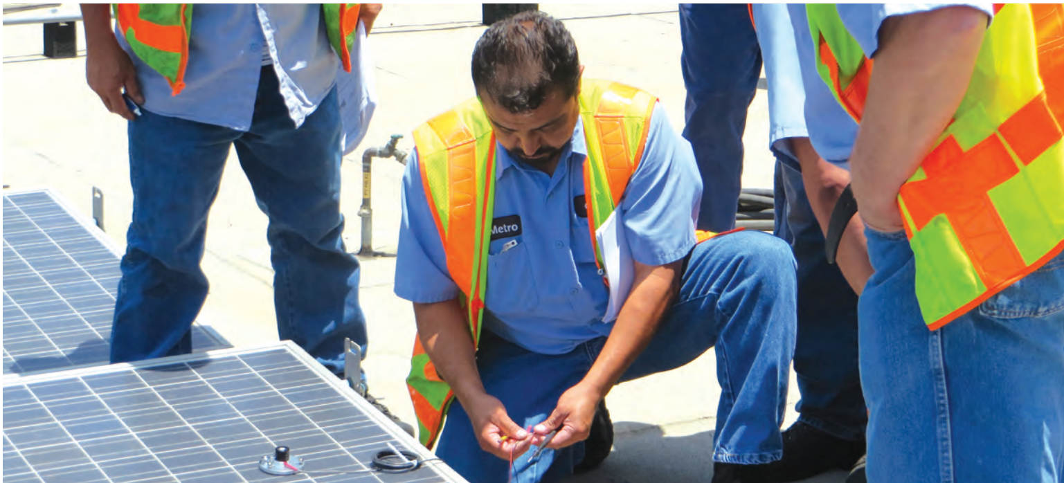
Metro staff conducting on-site PV maintenance training
