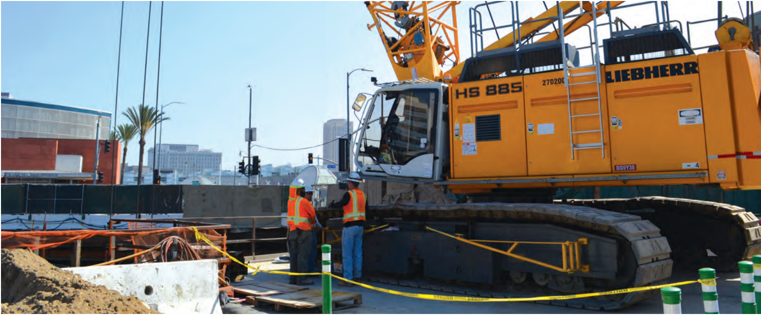
Construction equipment powered by renewable diesel in use at the Metro Regional Connector project
