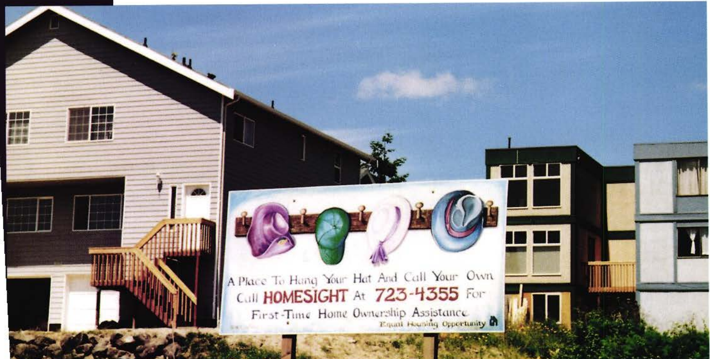
HomeSight, a non-profit housing corporation, builds housing on vacant lots turned over to the city of Seattle, WA, from WSDOT. The homes above are in Judkins Park.
