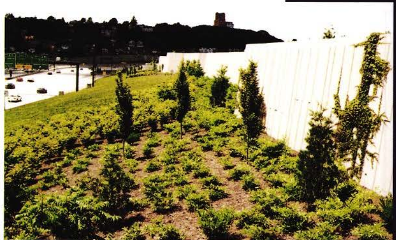
Noise barriers and outward-sloping buffers to reflect noise upward minimize noise impacts to the adjoining Seattle, WA, communities.
