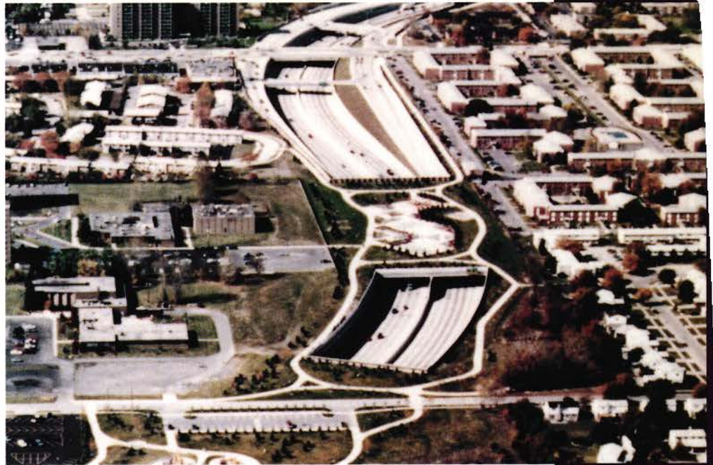
An aerial view of the two landscaped platforms over I-696 in Oak Park, MI. These decks provide pedestrian access and recreational areas for Oak Park residents.
