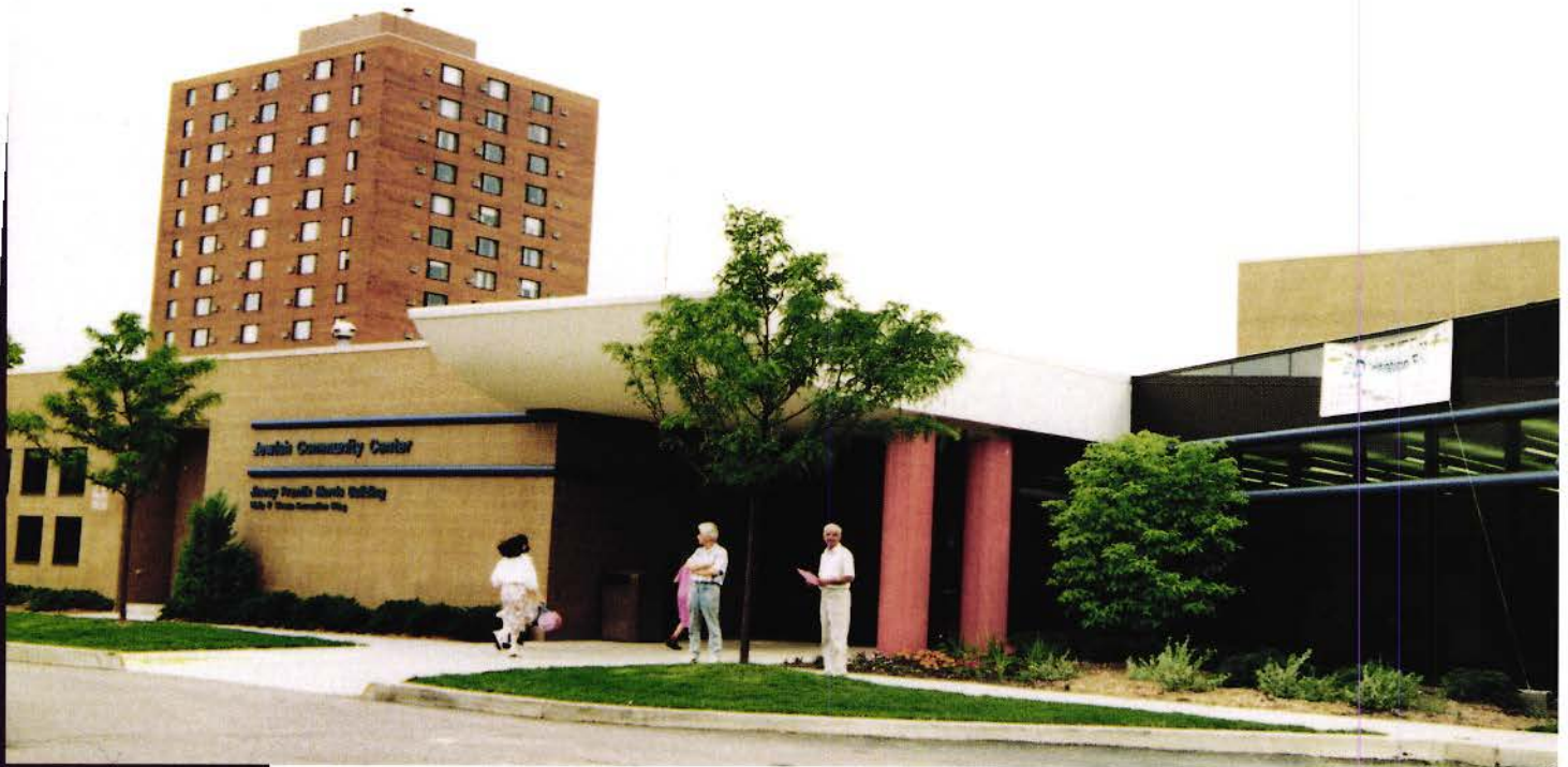
Two decks built over I-696 in Oak Park, MI, allowed fluid pedestrian movement across the freeway to shopping, synagogues, schools, and the Jewish Community Center (above).
