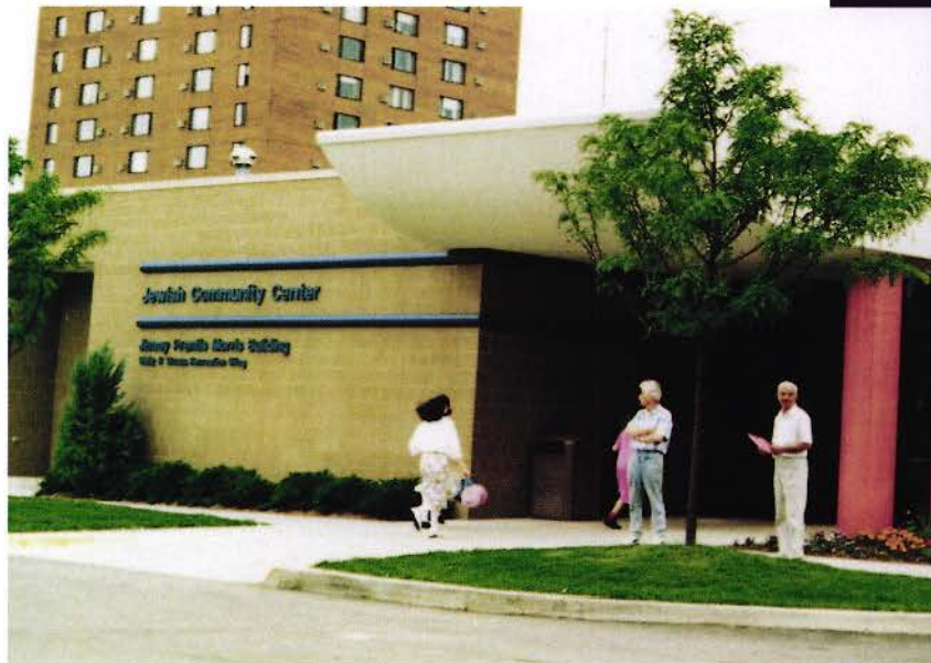
The Jewish Community Center (above) is an important public facility for the Jewish community of Oak Park, MI.
