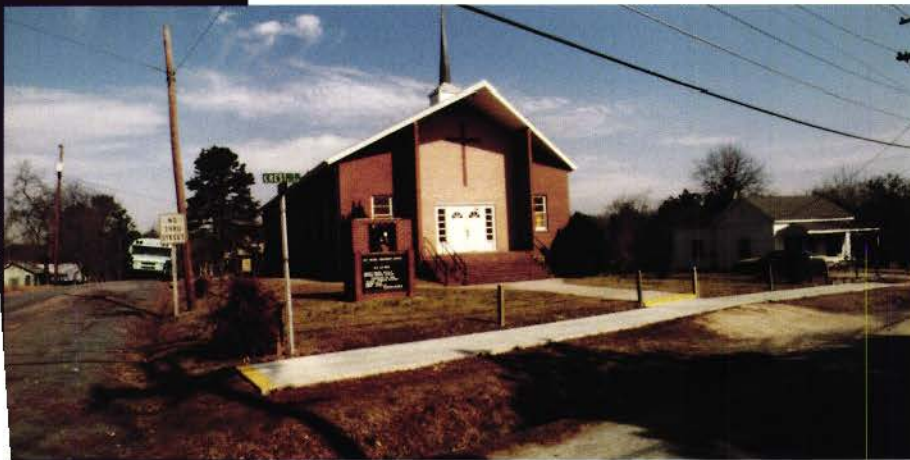
The New Bethel Baptist Church, built in 1965, was the focus of community life in Crest Street, Durham, NC. The church is shown as it was before the project.
