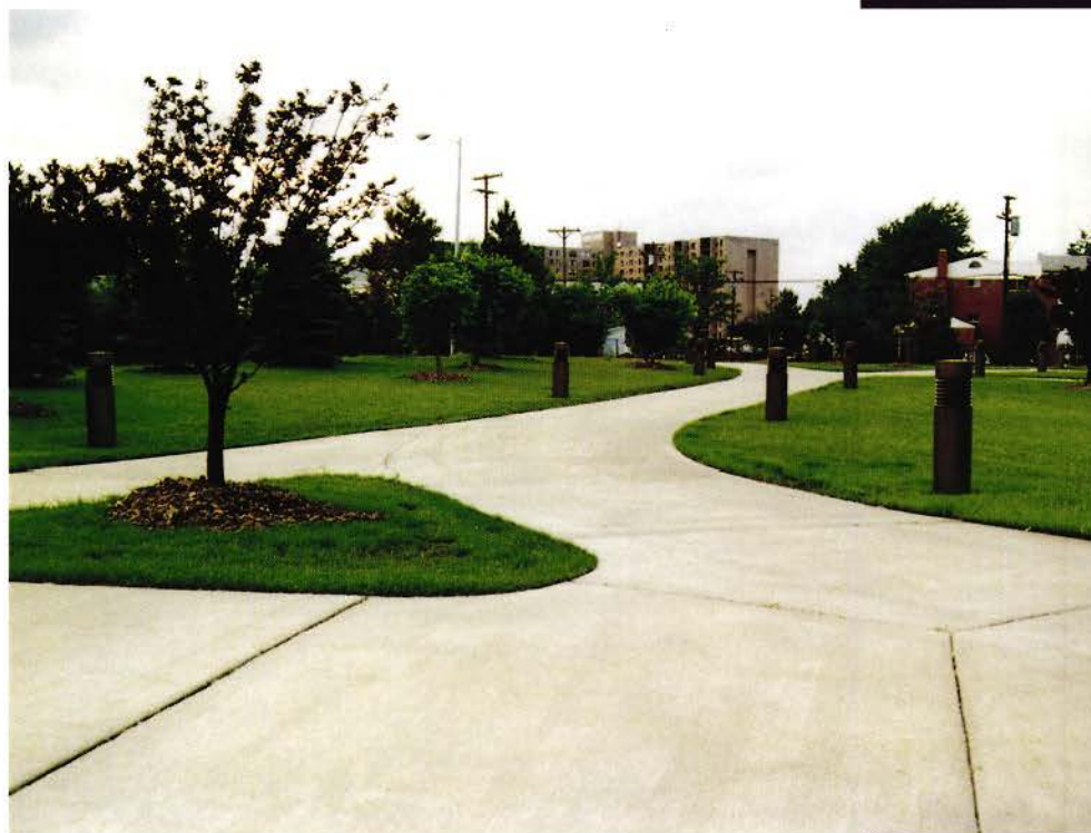
Paved and lighted pedestrian/bike paths alongside I-696 replaced informal, unlighted paths in use prior to the completion.
