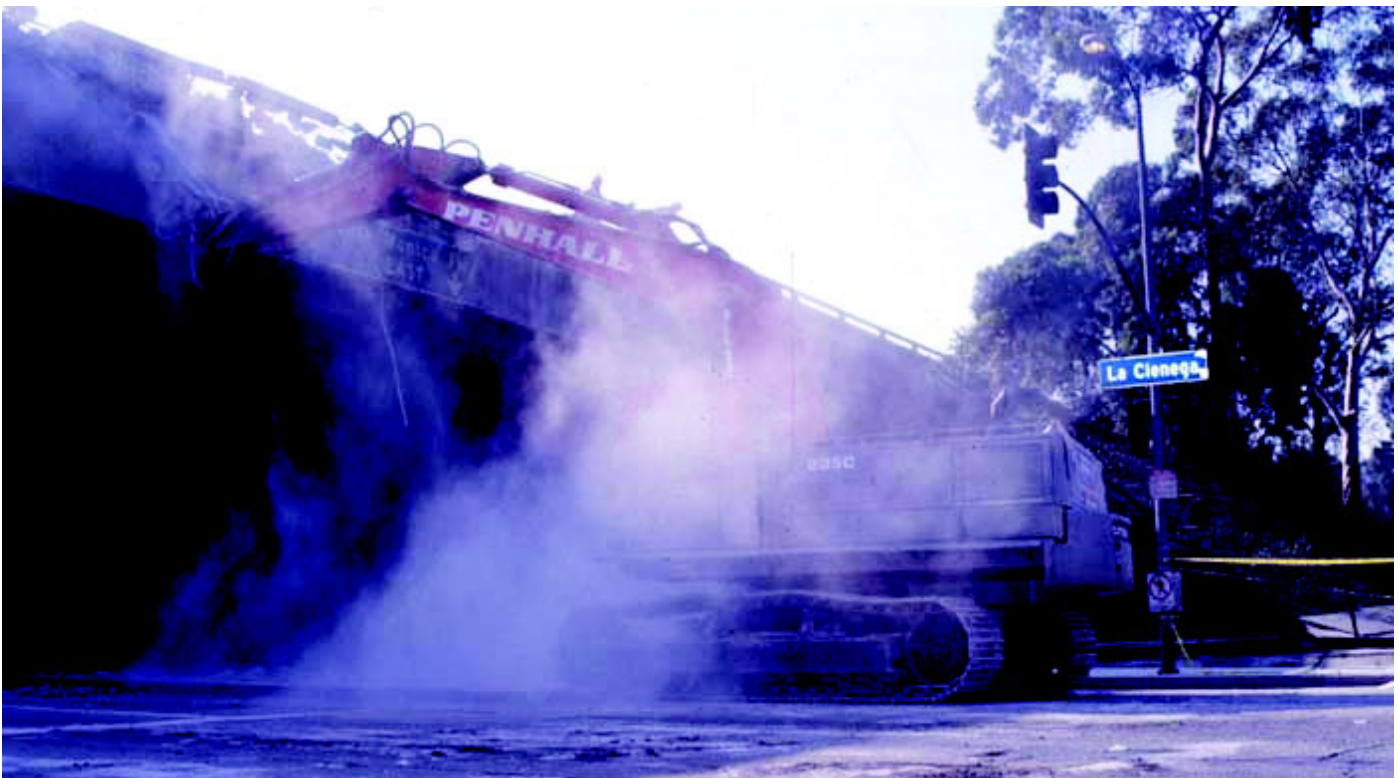
Figure 14. Demolition of I-10 at La Cienga Boulevard
