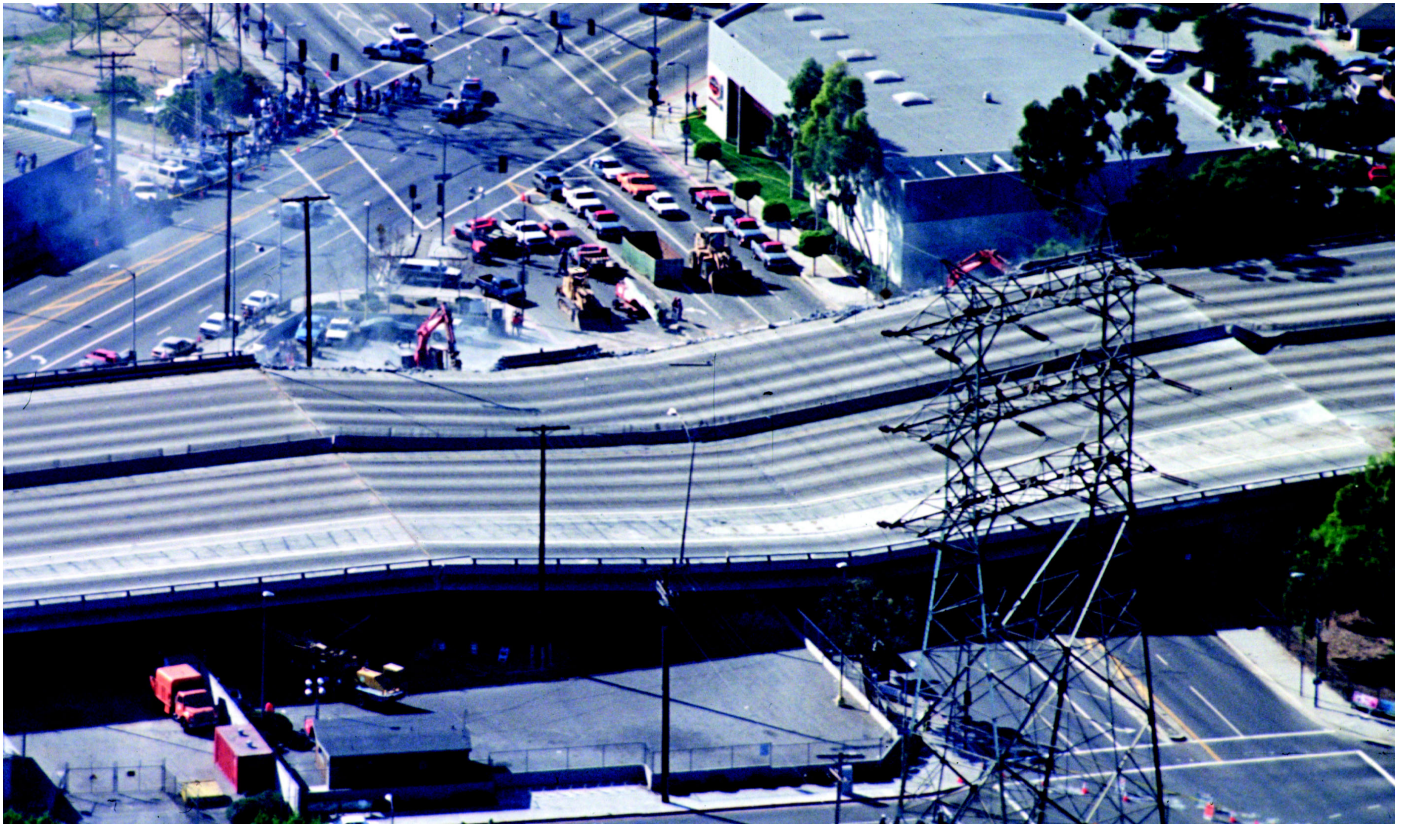
Figure 6. Damage at I-10/La Cienga Boulevard
