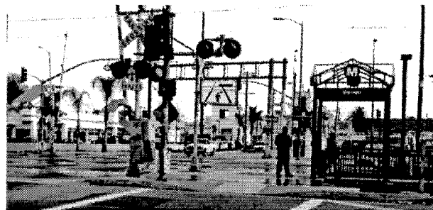
Exhibit 13 Fiber-optic active warning signs
