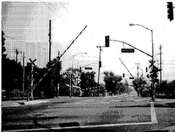
Exhibit 1 Typical quad gate at-grade crossing
