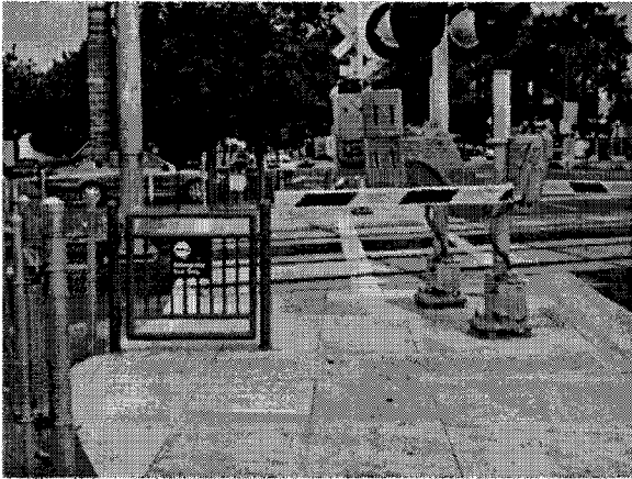
Exhibit 4 Emergency exit and pedestrian gate in down position. The yellow tactile strip alerts the visually impaired.
