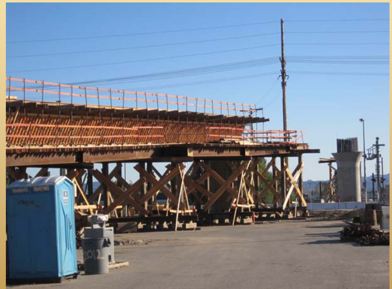
DWP Power Pole to be removed on Lassen Street
