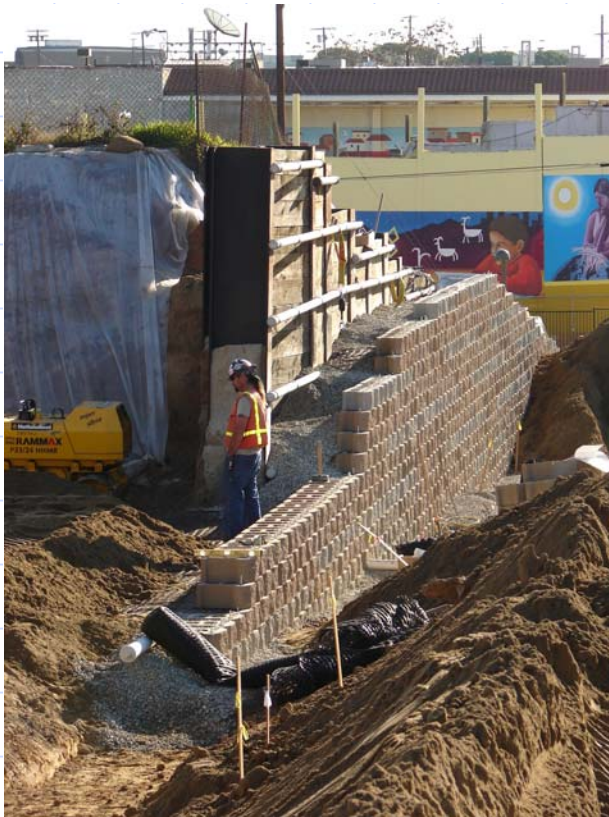
Construction of the retaining wall at the Northeast corner.
