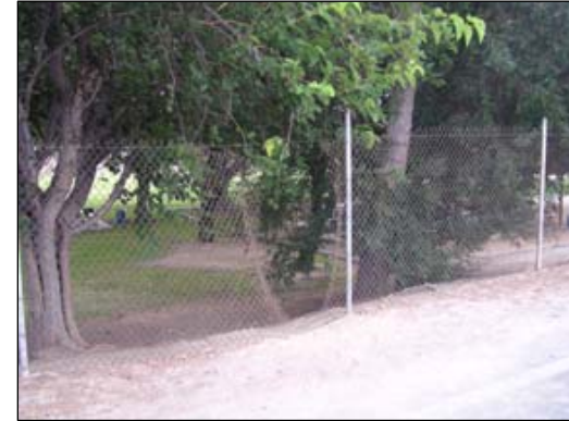
Cut fence along Rio Hondo bike path, showing desire for access to park
