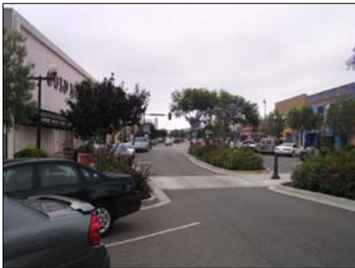
Facing north on Market Street
