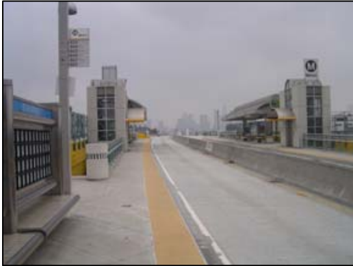
Harborway Transit Center at freeway grade
