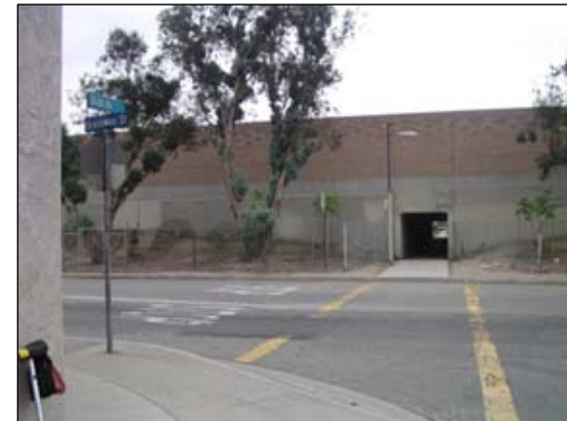
Pedestrian undercrossing at Utah Ave. and the 10 freeway
