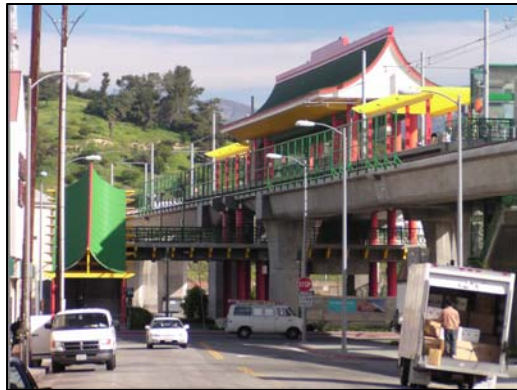
Spring Street facing north towards station
