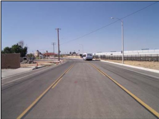
6 th Street East, facing north
