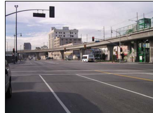
Alameda Street facing south across College Avenue
