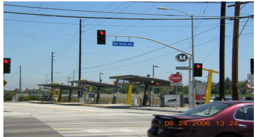
DeSoto-Phase IV (installation in progress)
