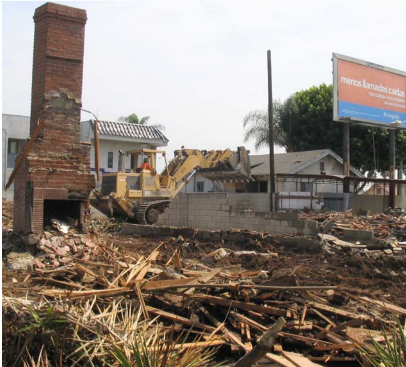
3 rd Street and Indiana Street Intersection
