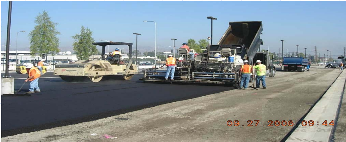
Parking lot paving operations
