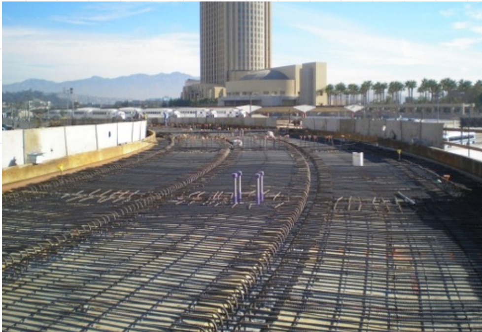
LRT Bridge Structure facing towards Union Station and Gateway Plaza.
