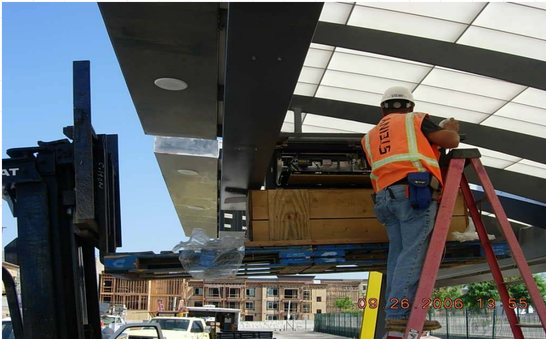
Installation of Variable Message Sign at station platform
