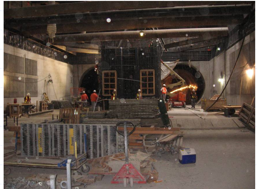
1 st /Soto Station – Work on the track level equipment rooms has begun.
