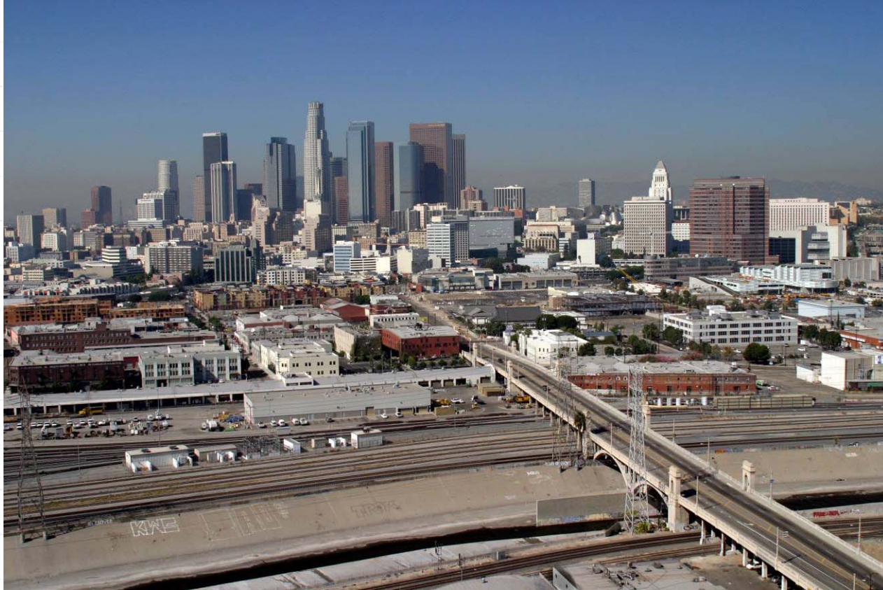
View of the LA River 1 st Street Bridge prior to bridge widening.
