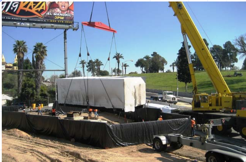
Traction Power Sub-Station 4 Installation
