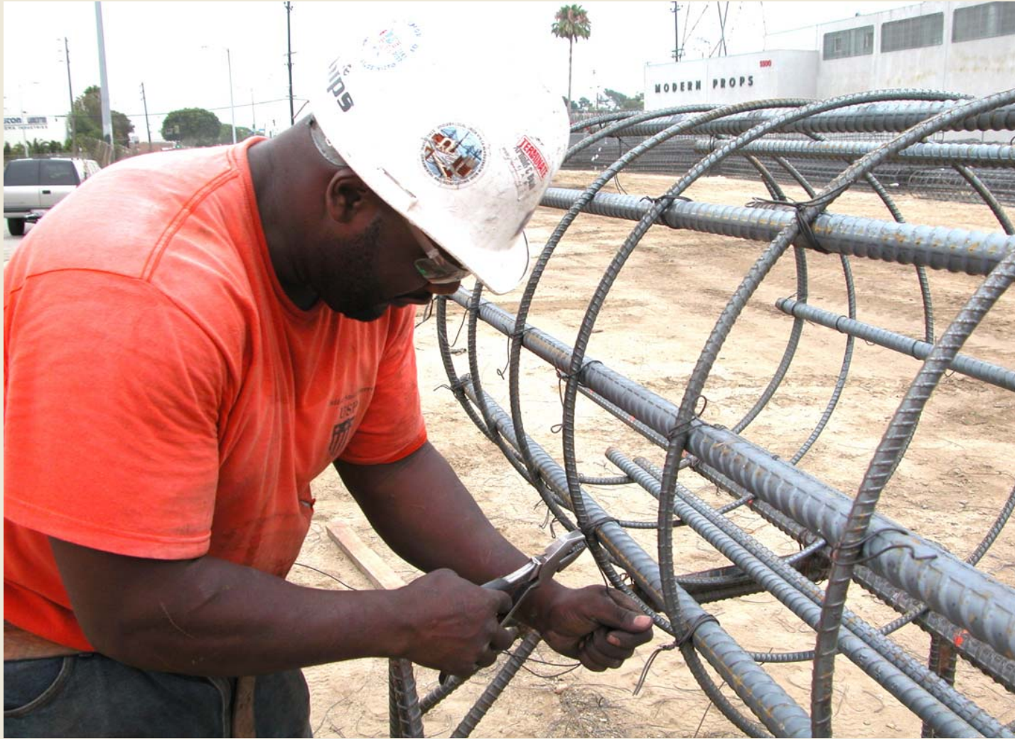
Tying Rebar Cages for CIDH Piles
