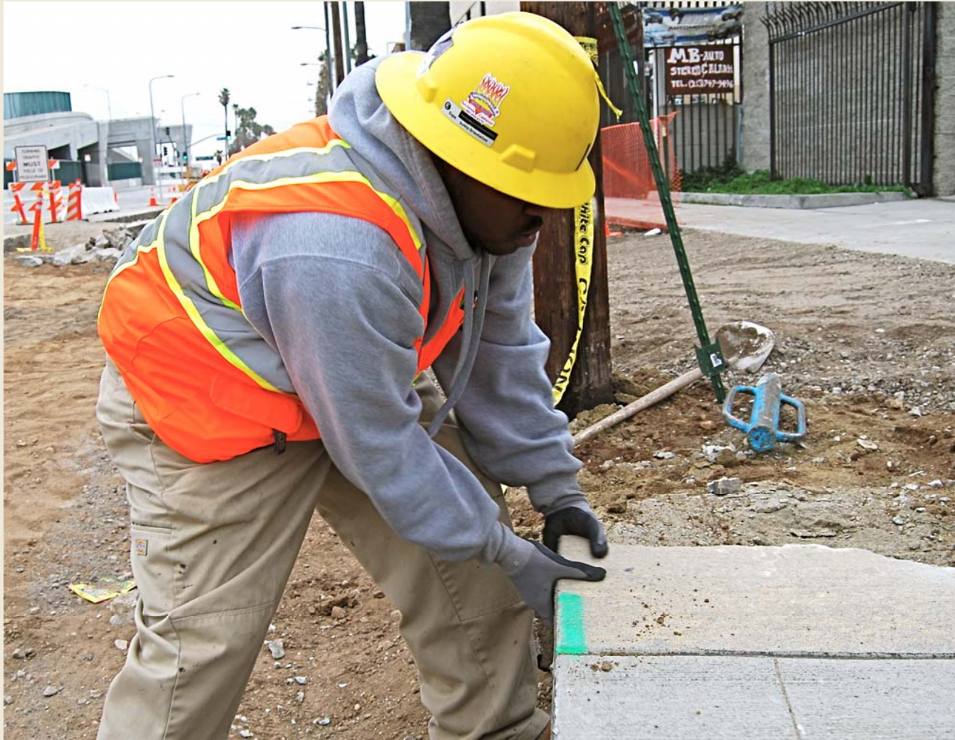
Demolition at Flower and Adams
