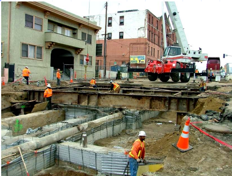
Deck beam removal along 1 st Street near Boyle Avenue.
