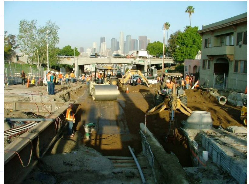
Earth backfill over underground structures.
