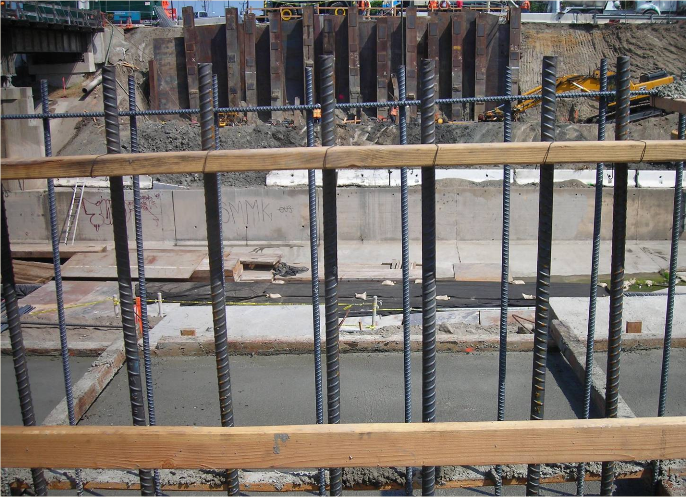
Abutment Wing Wall at National Blvd Bridge
