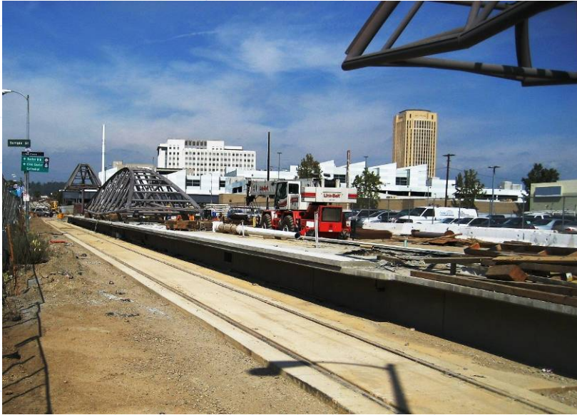
Little Tokyo/Arts District Station - Northeast corner of 1st/Alameda.
