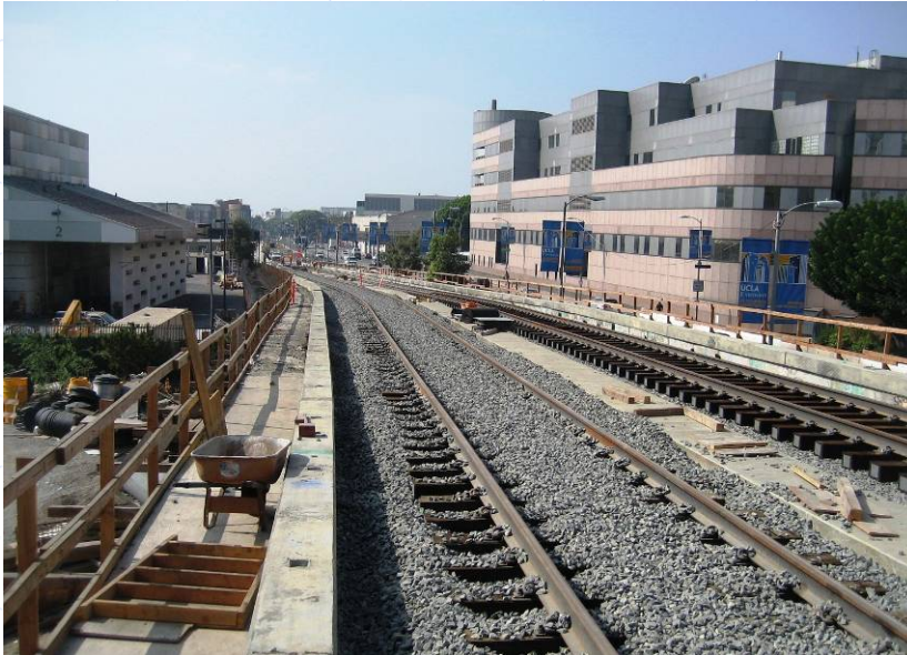
Trackwork and guideway construction from 1 st /Alameda to Union Station.
