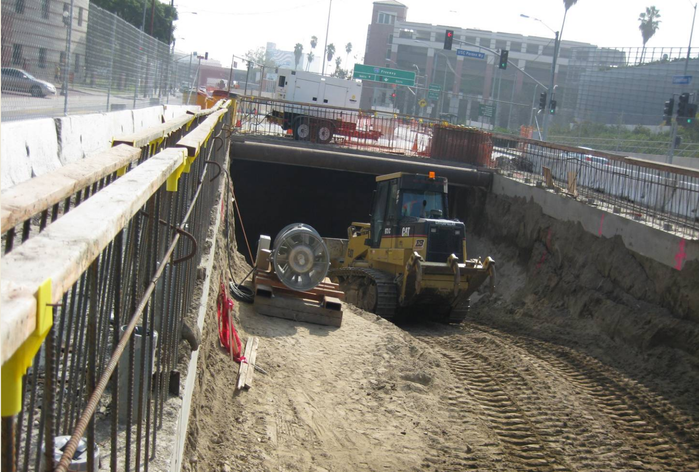
Began Excavation of Trench Structure
