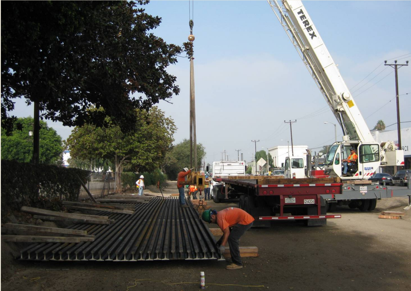
Began Receiving Running Rail
