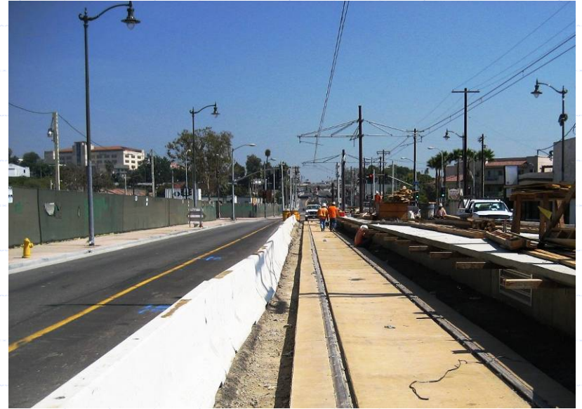
Pico/Aliso Station – View east near 1 st /Utah towards Boyle Heights.
