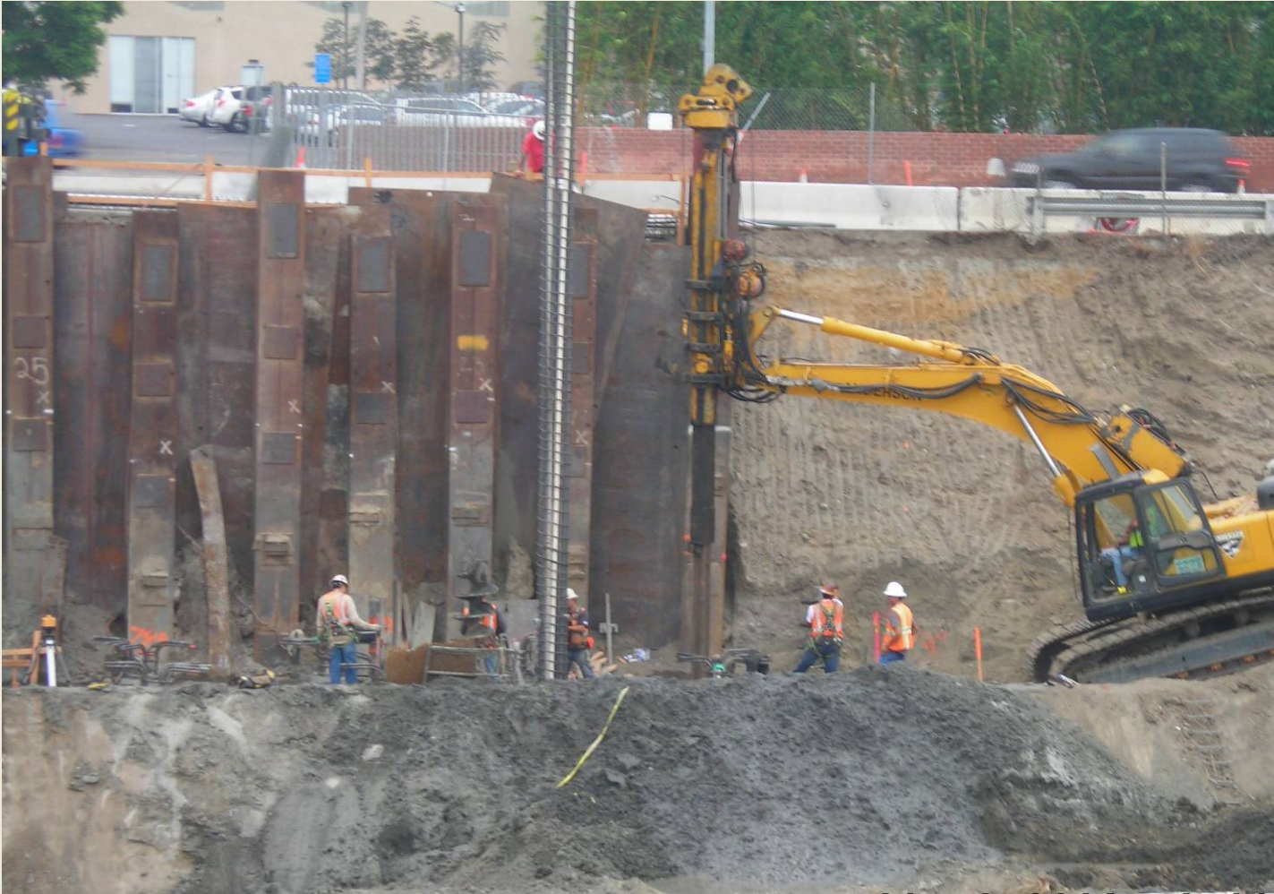
Abutment at National Blvd Bridge
