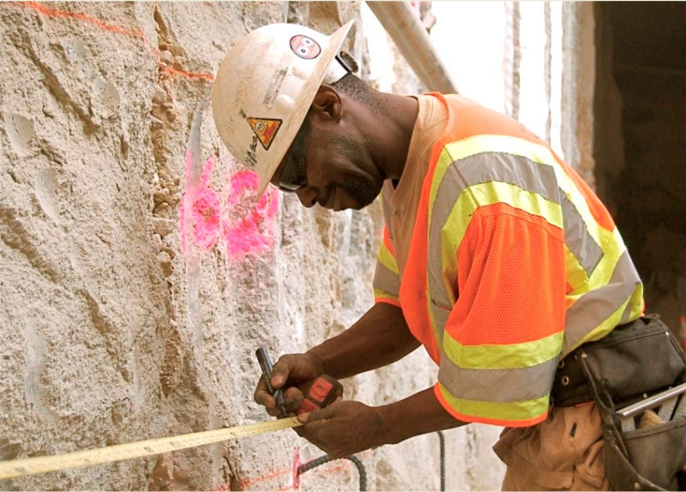
Preparation for drilling of dowels at A3 Trench walls
