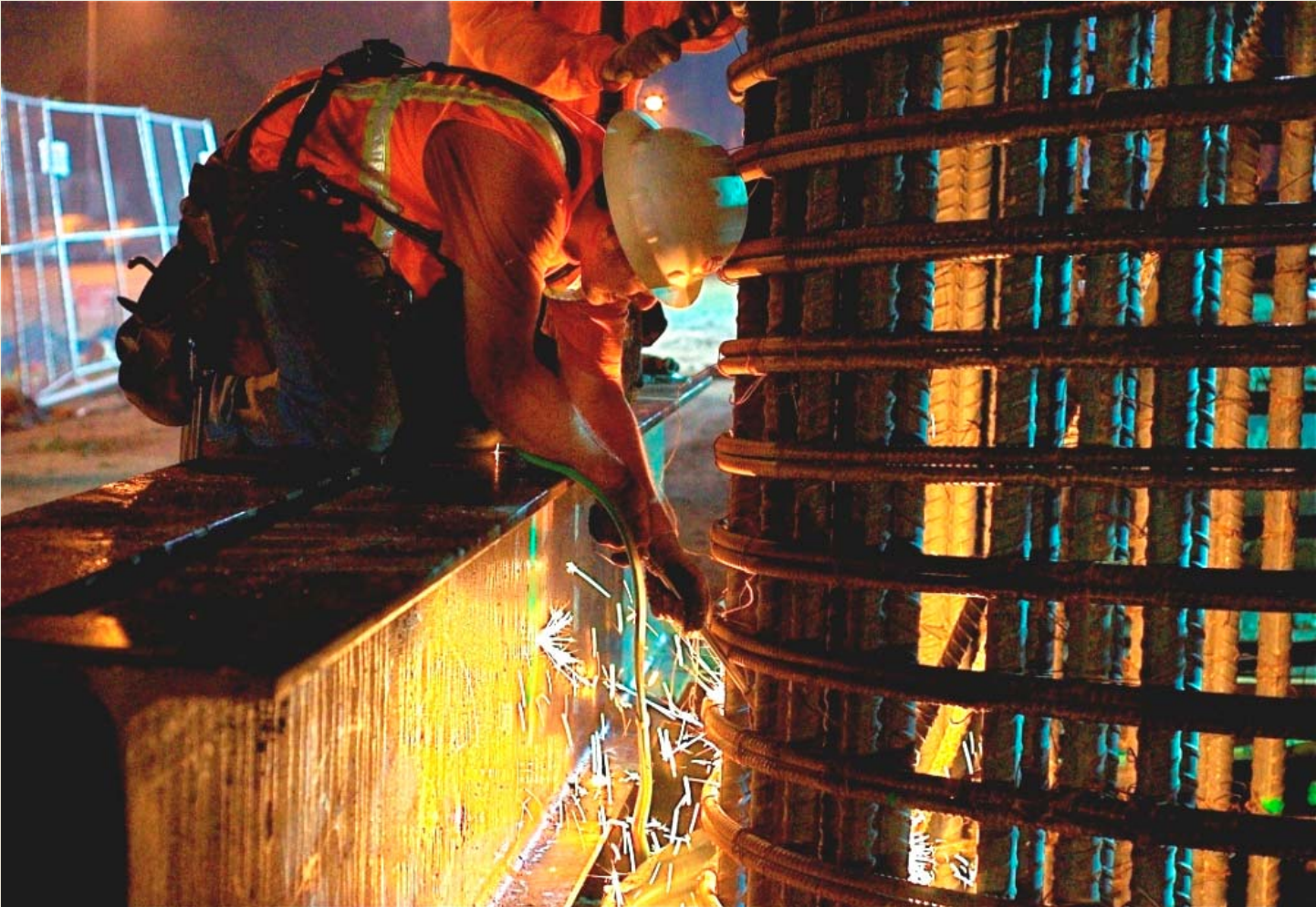
Completing the 11' CIDH piles for La Cienega overcrossing
