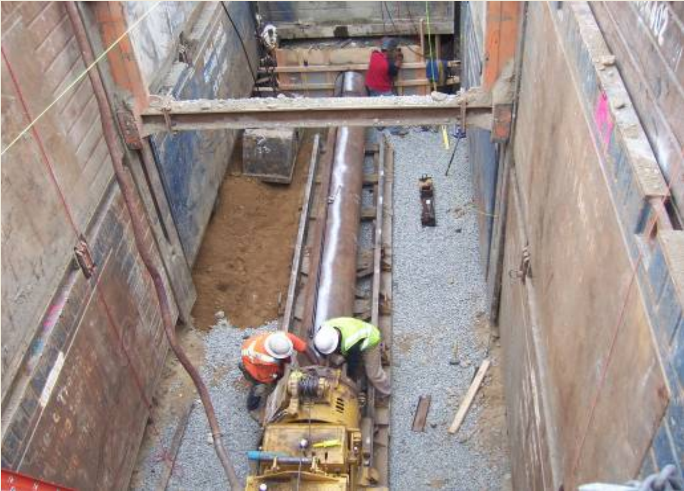
Boring for Ductbank Conduits at Arlington Ave. and Exposition Blvd.
