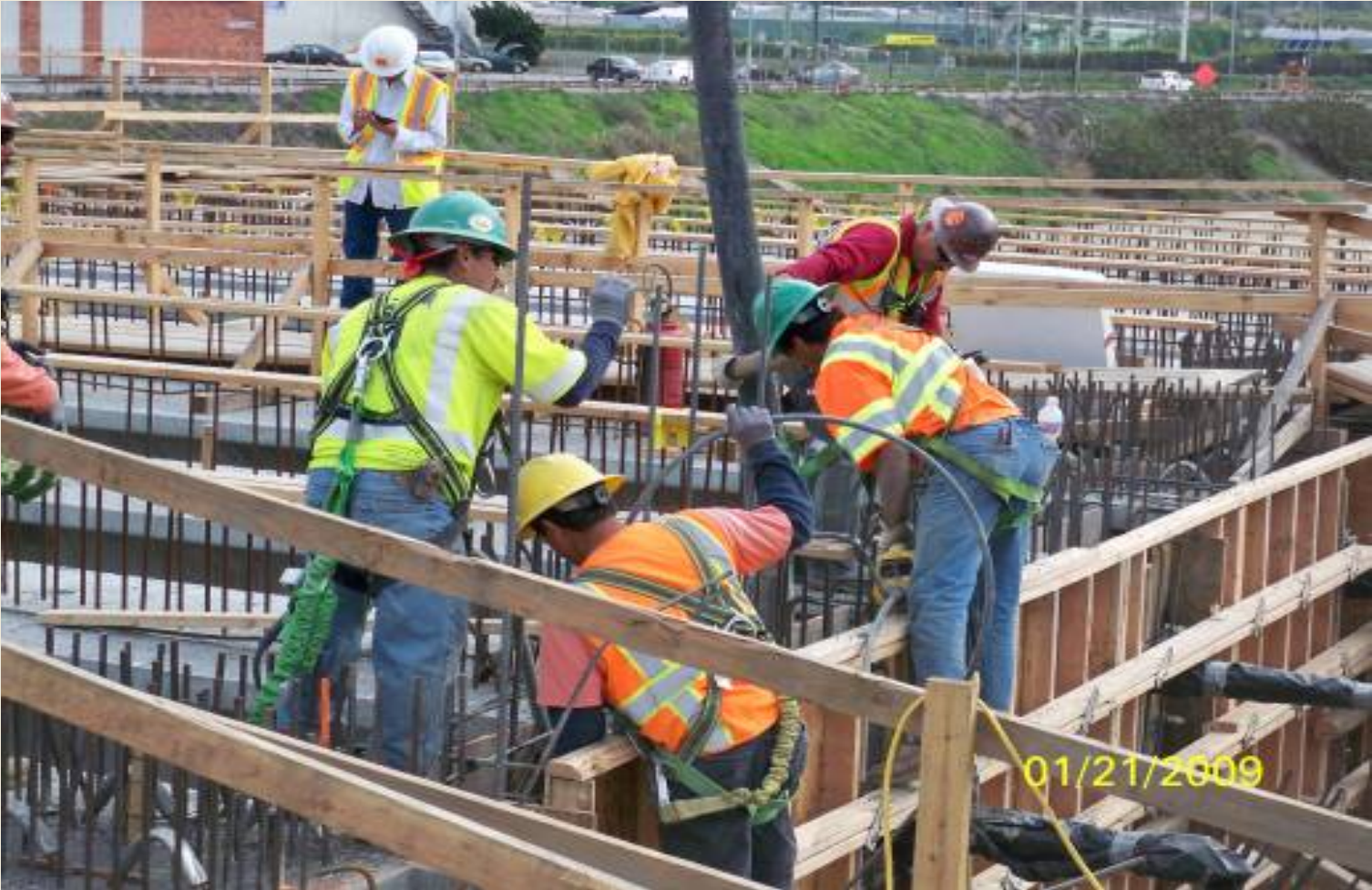
Concrete Placement for End Diaphragms at National Boulevard Bridge
