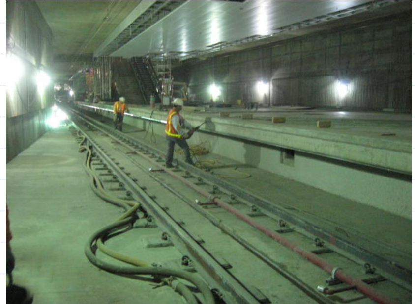
Installation of floor finishes continues on the train passenger platform.
