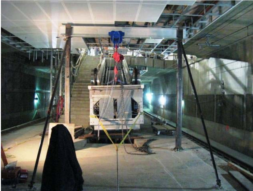
Escalators and elevators are being installed along with architectural finishes.
