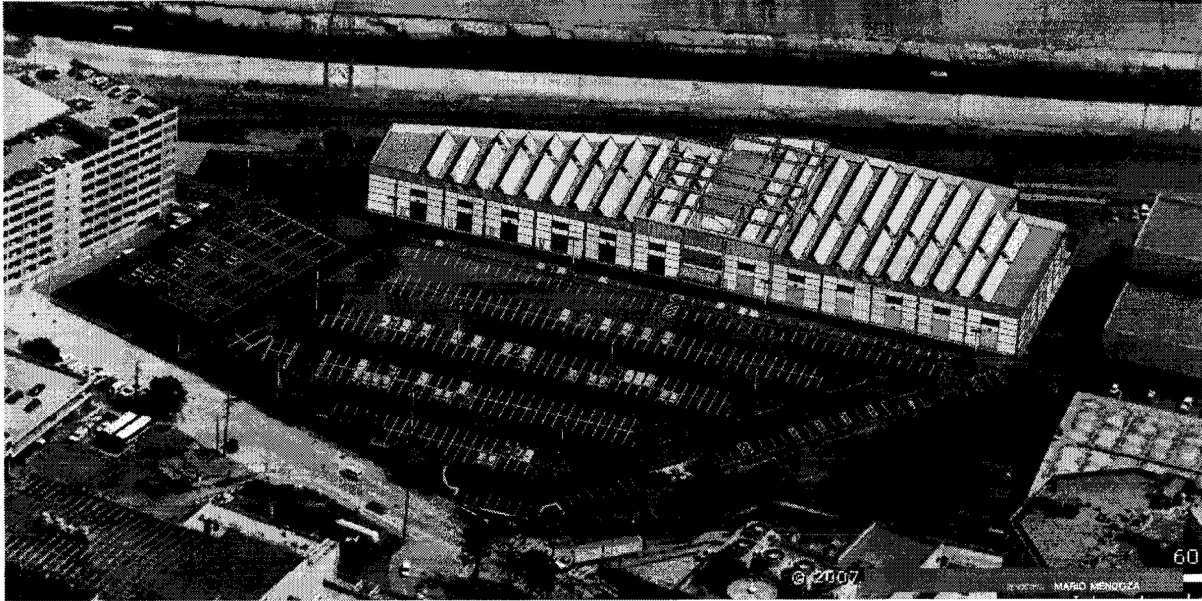
BAUCHET STREET STORAGE AND FACILITIES MAINTENANCE STRUCTURE
