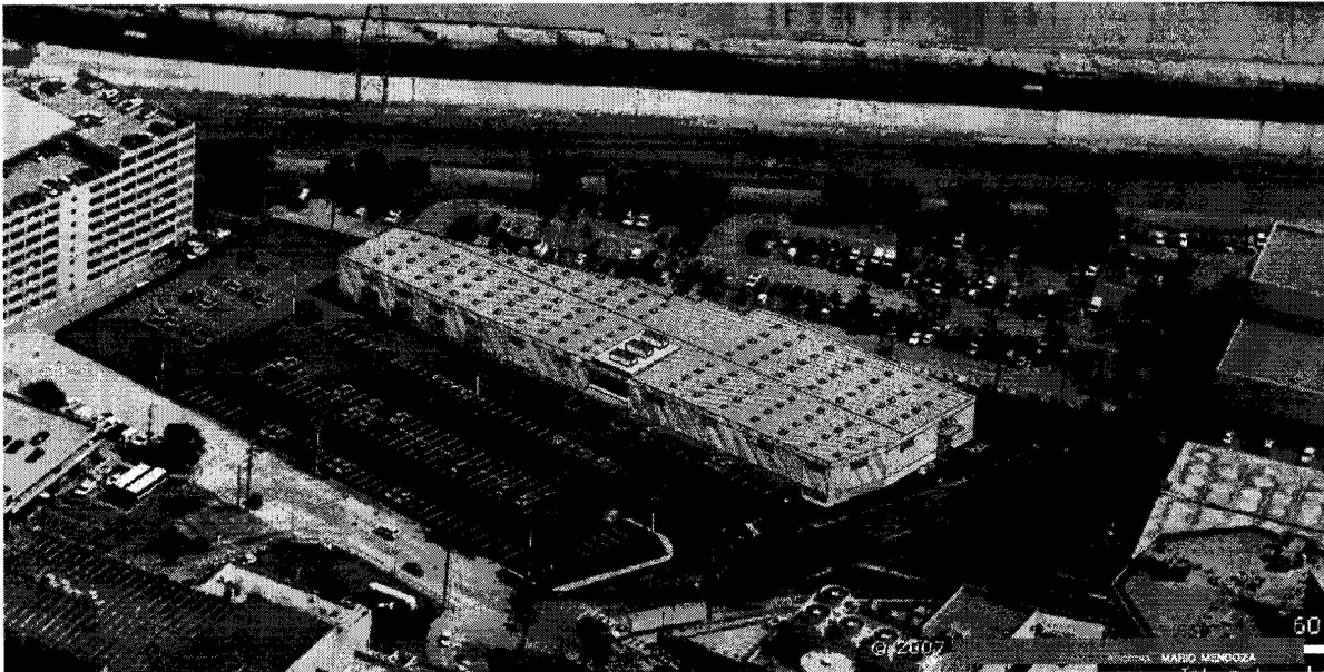
BAUCHET STREET STORAGE AND FACILITIES MAINTENANCE STRUCTURE
