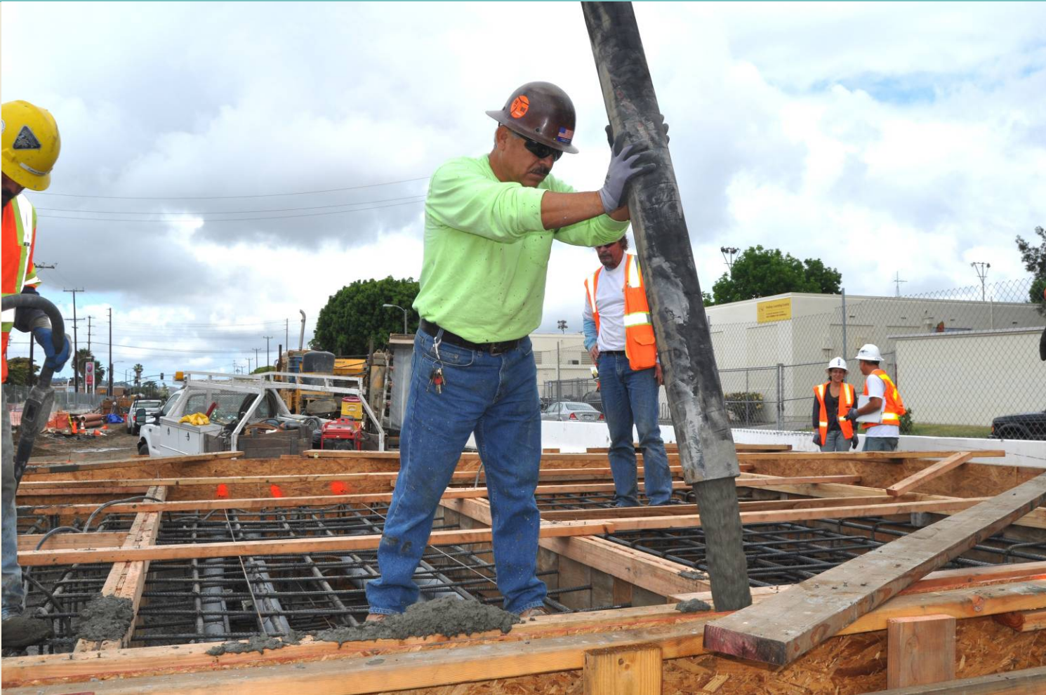
Concrete Pour for Approach Slabs at Harvard Pedestrian Crossing Tunnel
