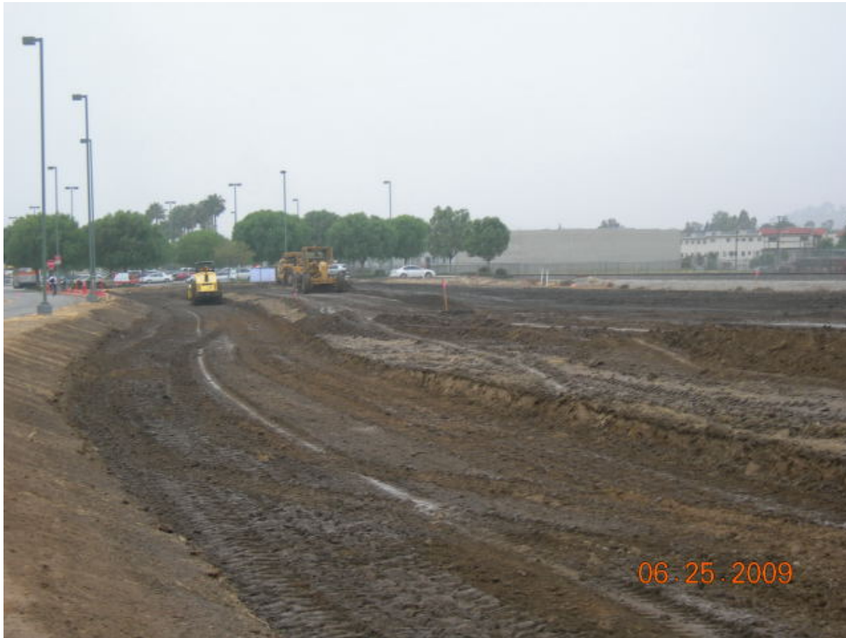
Construction begins at North Parking Lot
