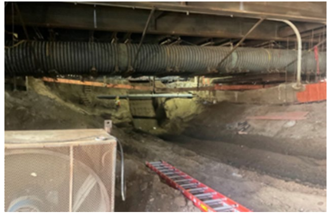
Westwood/UCLA Station: Station Box Excavation and Utility Supports Underneath Wilshire Blvd
