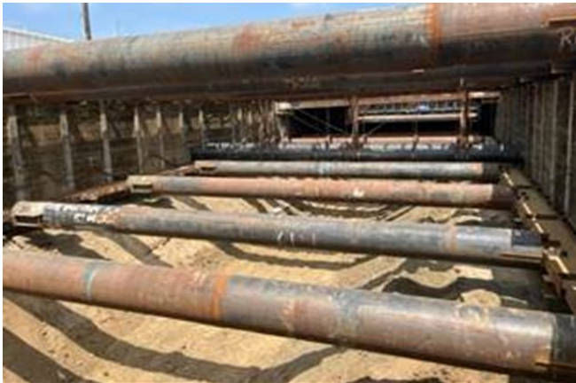
Westwood/VA Station: Installation of Level 2 Struts Between GL22 & GL01
