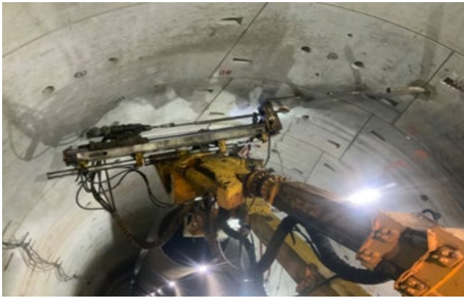
BR Tunnel – CP-55 Tube Spile Installation
