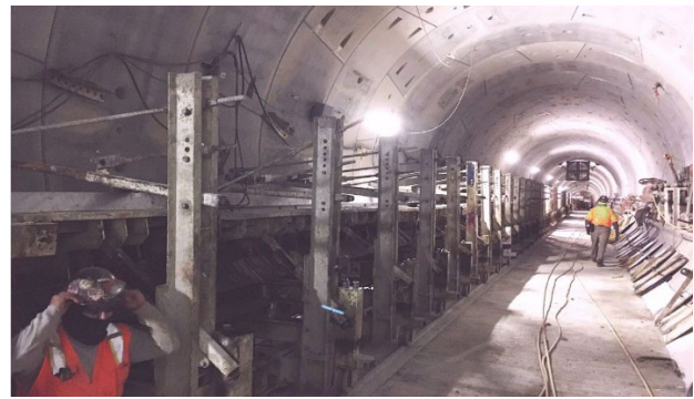
Reach 4 (BR) Walkway Construction
