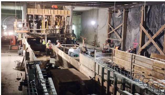
Platform Construction at Wilshire/Fairfax Station
