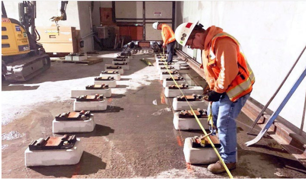
Track Installation at Wilshire/Western Interface Chamber
