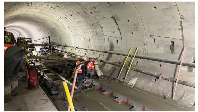
Reach 3 (Fairfax – La Cienega) Track Infill Slab Placement
