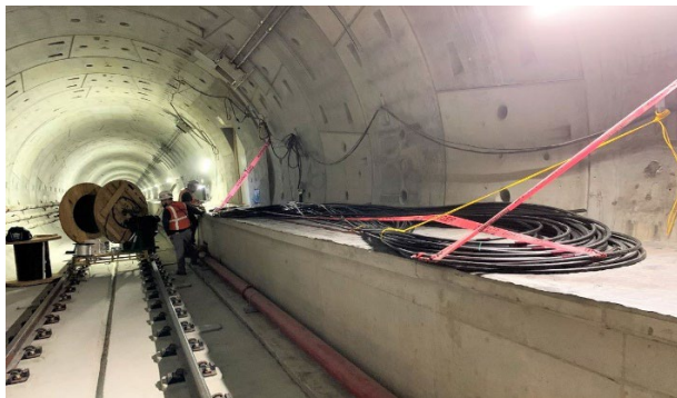
Reach 2 (La Brea - Fairfax) Communications Cable Installation
