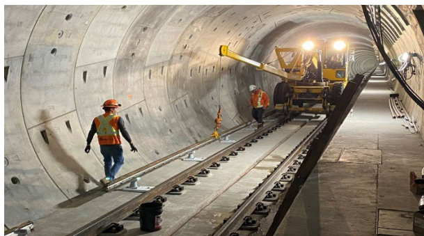
Reach 1 (Western – La Brea) Third Rail Installation
