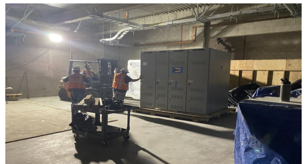
TPSS Equipment Installation at Wilshire/La Cienega Station
