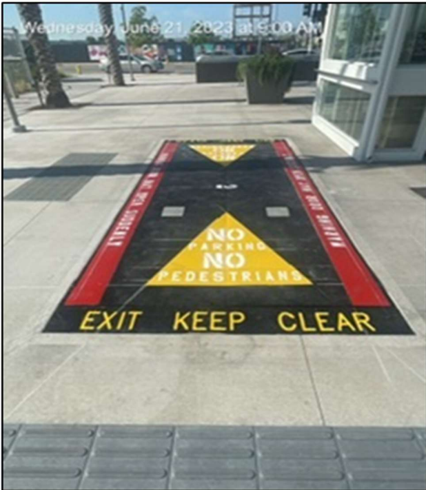
Expo Station: Falcon Striping Co. painted emergency hatch covers.
