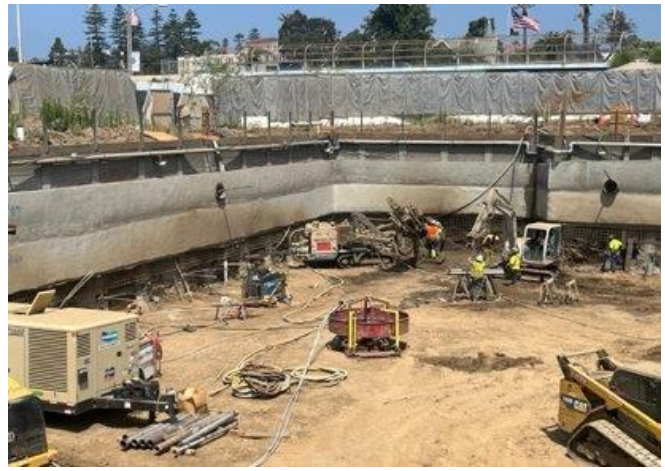
Installation of Level 2 Tiebacks & Shotcrete at the Westwood VA Station Entrance
