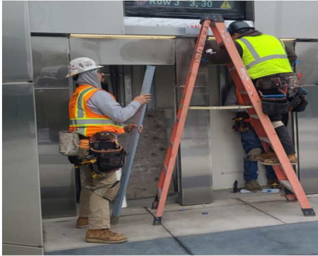
Stainless steel cladding installation around TVM at Little Tokyo/Arts District Station
