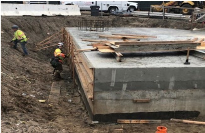
VA Steam Tunnel – Roof Installation on Vaults 200 & 300
