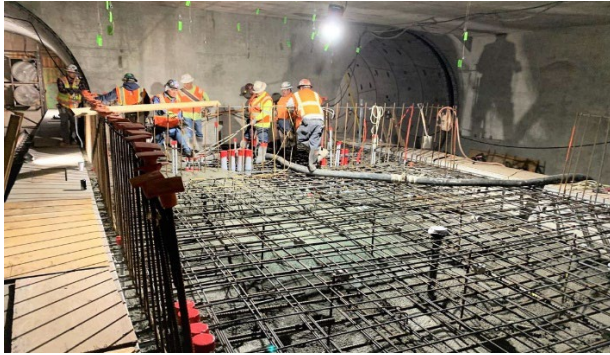
Room Slab Placement at Western Interface Chamber
