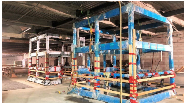
Elevator Frame Installation at Wilshire/Fairfax Station
