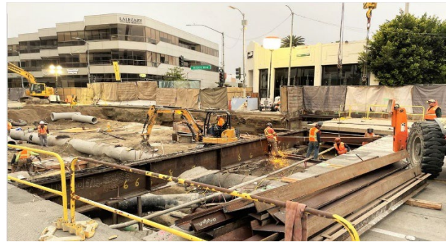
Weekend Decking Removal at Wilshire/La Cienega Station
