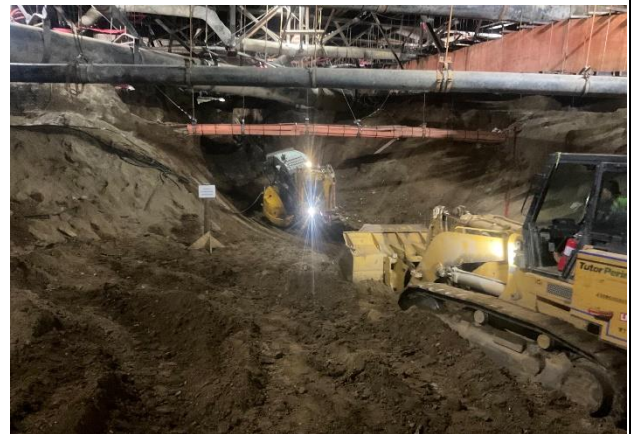
Westwood/UCLA Station: Station Box Excavation and Utility Supports
