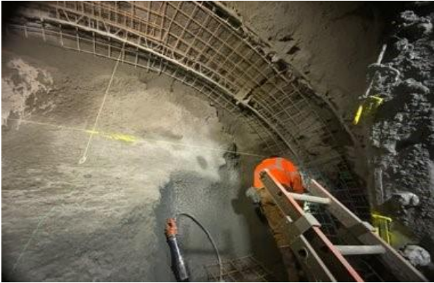
BR Tunnel at CP-55 Shotcrete/lattice girder installation
