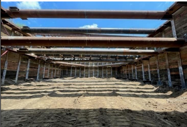
Westwood/VA Station: Installation of Level 3 Struts Between GL22 & GL01
