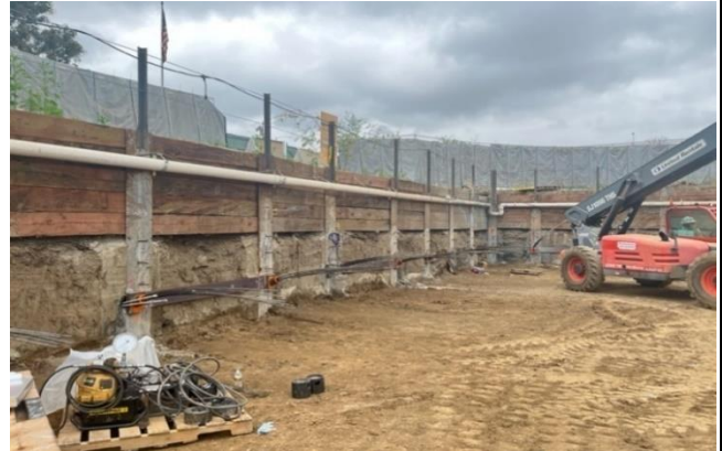
Installation of Level 1 Tiebacks at the Future Station Entrance
