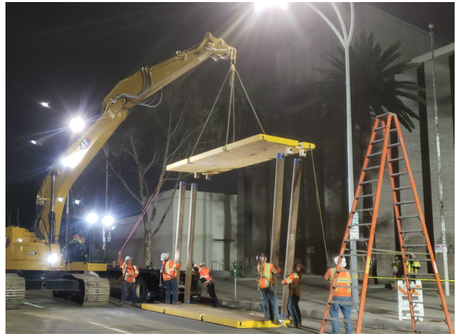
Assembling shoring box for Vault 6900
