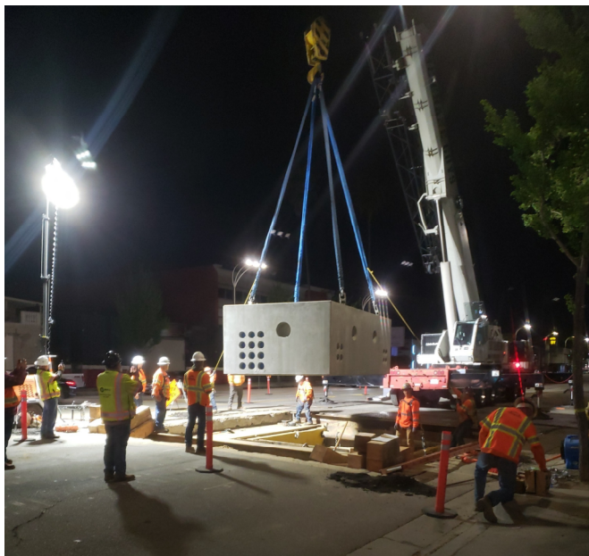
Installation of the upper portion of the vault
