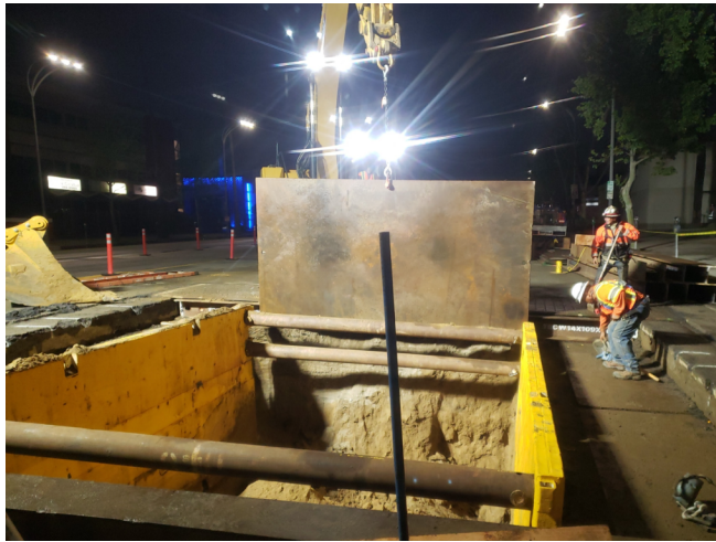
Trench shoring for Vault 6900
