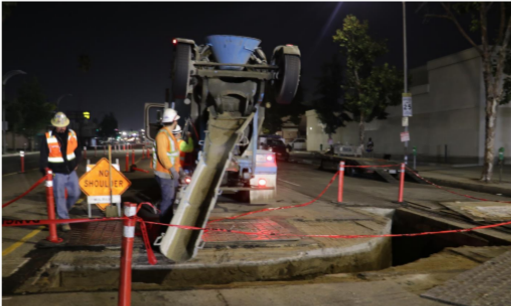
Slurry placement at lateral 06
