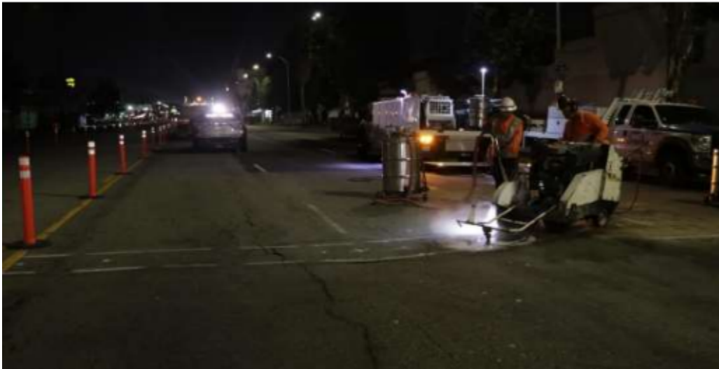
Tom Grabavac crew: Sawcut lateral 06
