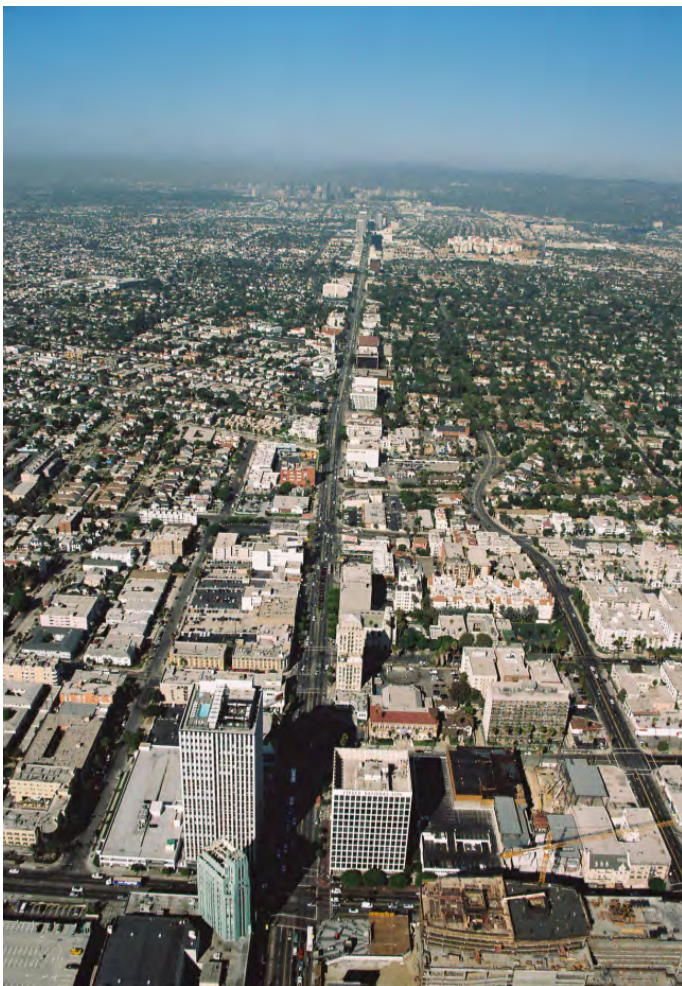
Figure 2-1. Wilshire Boulevard Corridor looking West from Western Avenue
