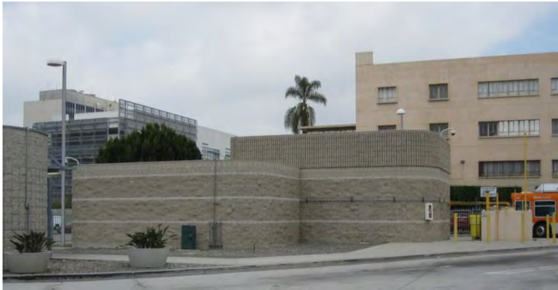
Figure 2-64. Existing Emergency Generator Structure at Wilshire/Vermont Station
