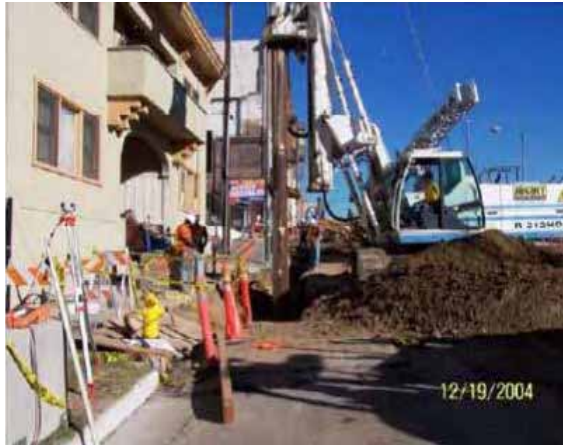
Figure 3-7: Pre-augering for Soldier Pile
