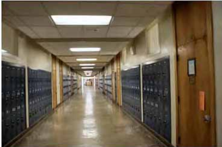
Figure C-9: Building B—Interior Corridor
