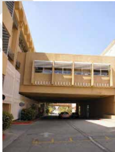
Figure C-14: Walkway from Building A over Heath Avenue
