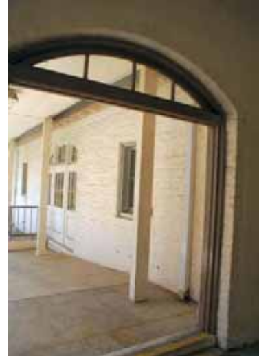
Figure C-10: Building B Interior
