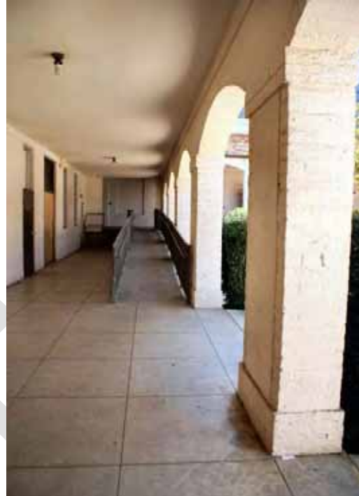
Figure C-8: Courtyard Columns in Building B
