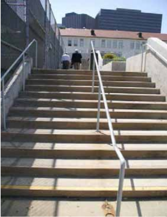
Figure C-7: Pathway leading to Building B
