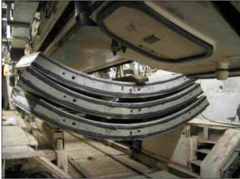
Figure 5-5: Double-Gasketed Segments at Tunnel Heading
