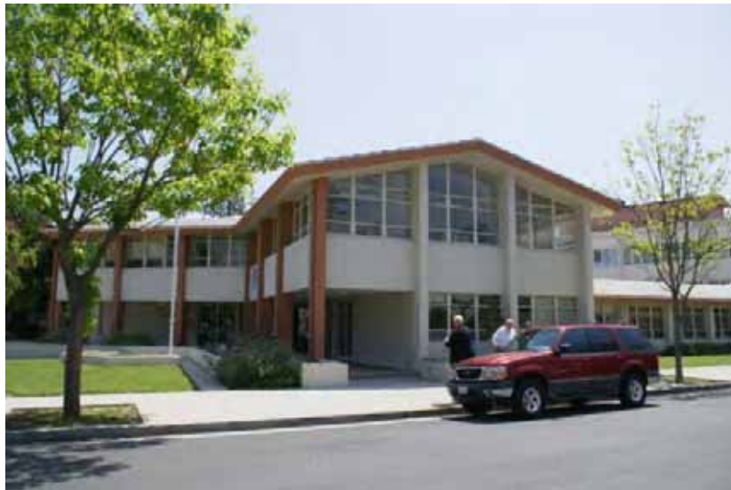
Figure C-1: Administration Building—Steel Framed Structure—Built in 1960s
