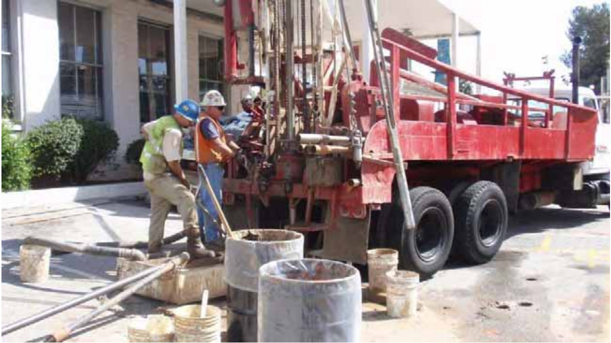
Figure 8-3: Drill Rig Outside BHHS Classroom Building
