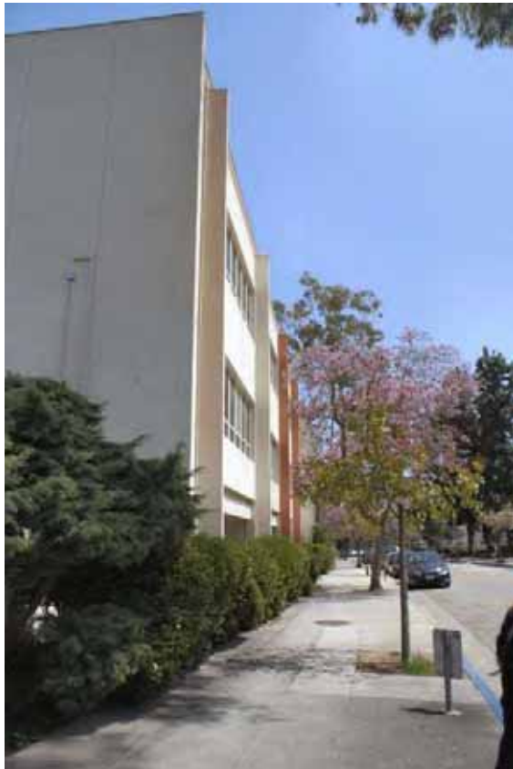
Figure C-3: Frontage of Instructional Center
