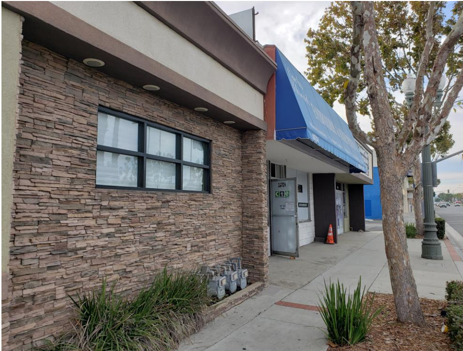
Photograph 2. Detail of façade, view to southeast, November 5, 2020
