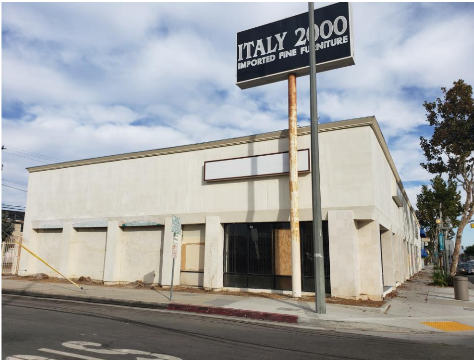
Photograph 2. South elevation, view to north, November 5, 2020
