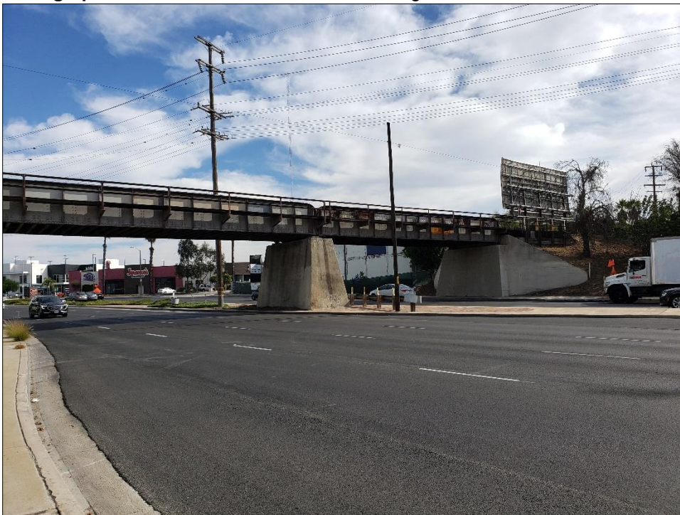
Photograph 3. Harbor Subdivision – Hawthorne Boulevard Bridge, view to northeast, November 5, 2020.
