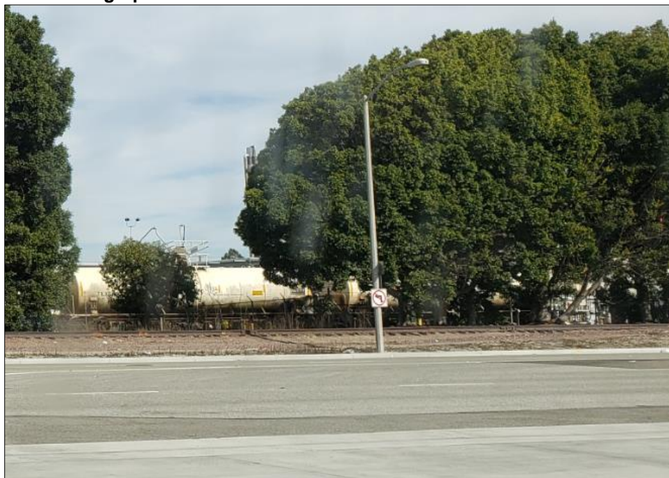
Photograph 1. View of Alcoa Spur Tracks from W Del Amo Boulevard, view to north, November 5, 2020.
