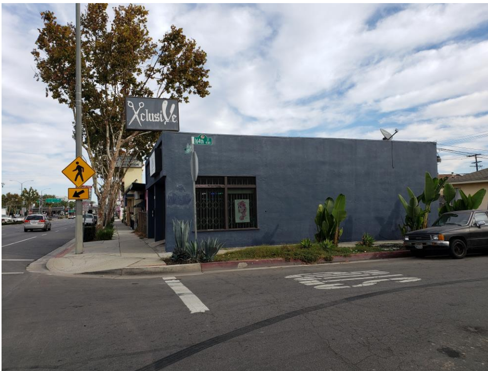
Photograph 2. South elevation, view to north, November 5, 2020
