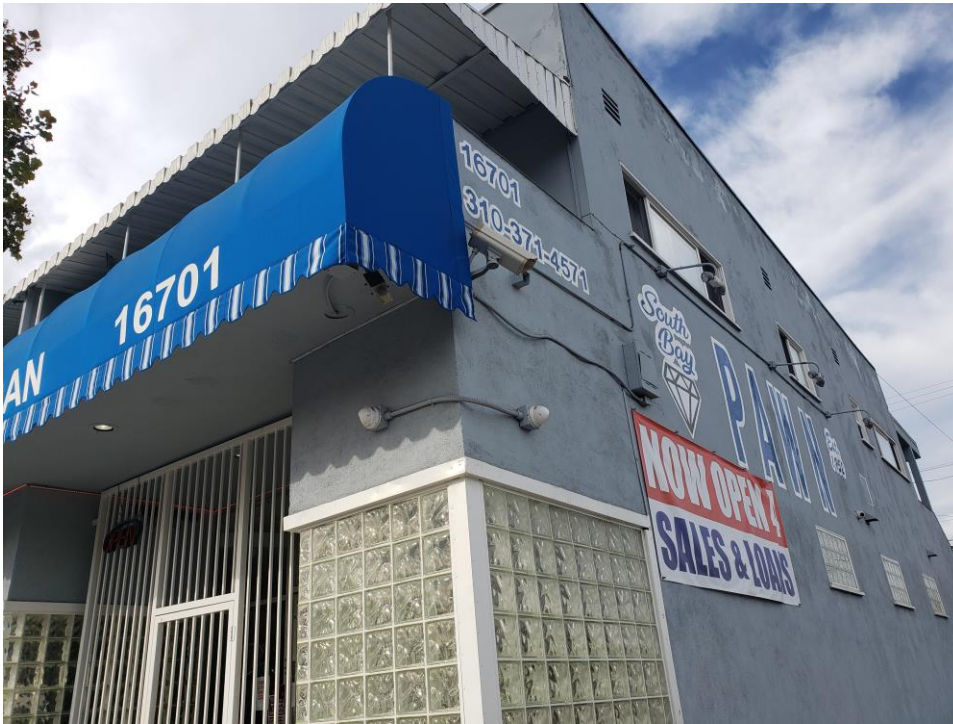
Photograph 2. East and north elevations, view to southwest, November 5, 2020
