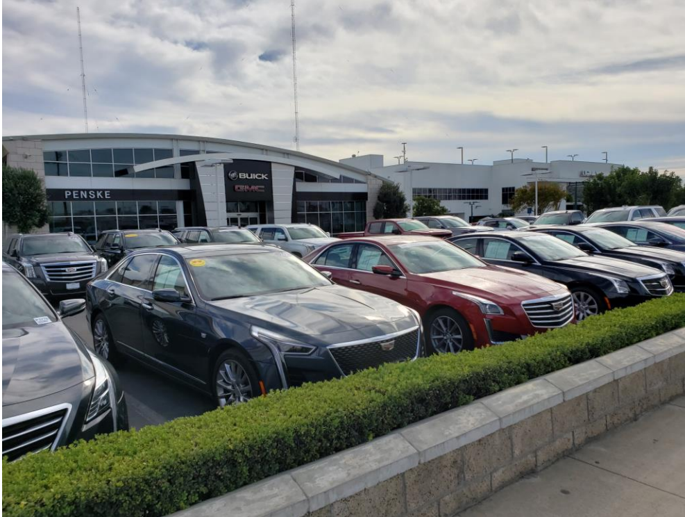
Photograph 2. West elevation, addition, view to southeast, November 5, 2020
