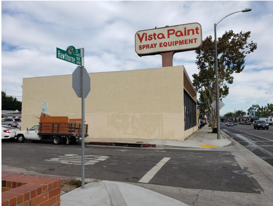
Photograph 2. South elevation, view to north, November 5, 2020
