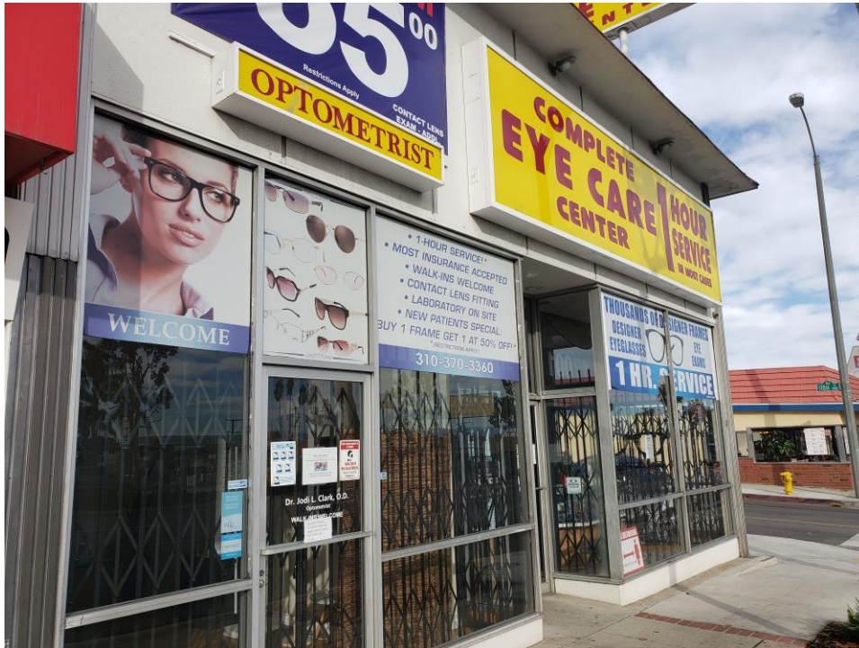
Photograph 2. Detail view of façade, view to northwest, November 5, 2020
