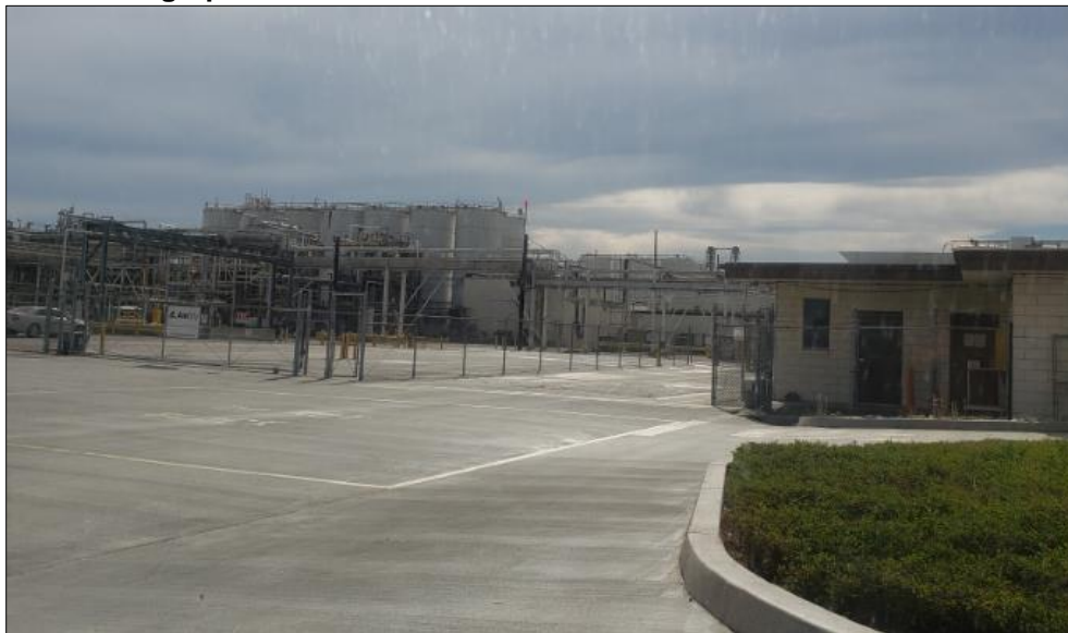
Photograph 1. Dow Chemical Plant, 305 Crenshaw Boulevard, Torrance, November 5, 2020.
