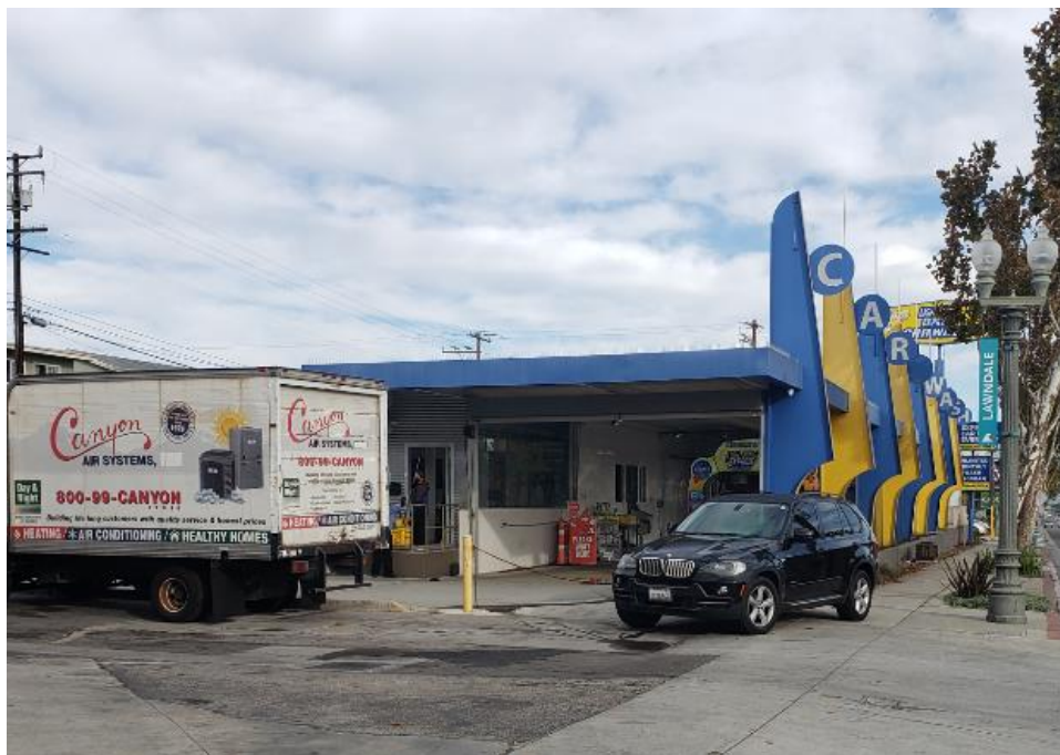
Photograph 2. South elevation, view to north, November 5, 2020
