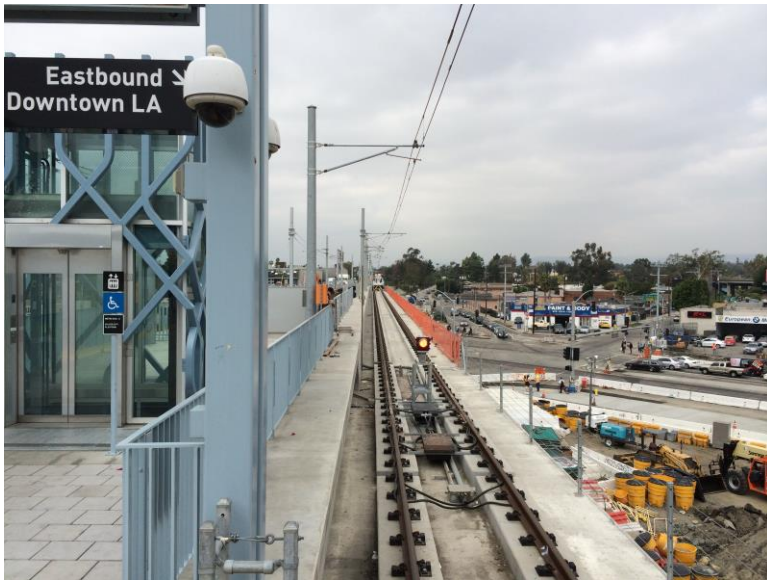
View of tracks looking west after tie-in work completion
