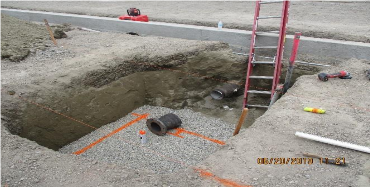
LEIMERT PARK STATION- Continued tile grout from mid landing to plaza at entrance stairs #1.
