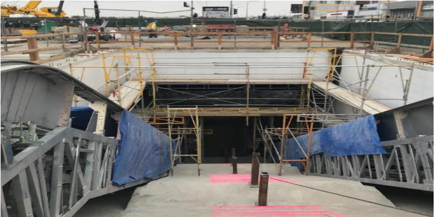
EXPOSITION/CRENSHAW STATION – Continued tile installation from mid landing to plaza.
