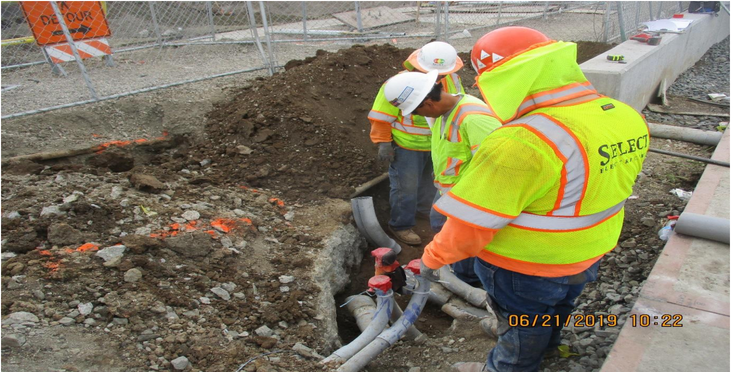
FLORENCE/CENTINELA - Select Electric Place conduits and pull boxes at Centinela and Florence crossing.
