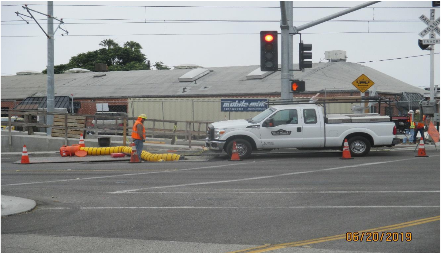
FLORENCE/CENTINELA - Stripping and grouting the manhole on Florence.
