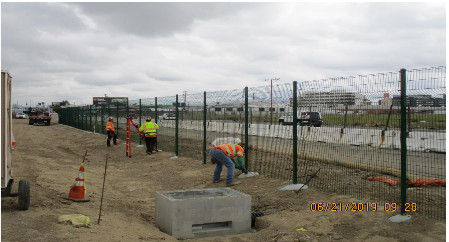
UG-1- A Guideway between UG1 and 104th St. wire fence placement.
