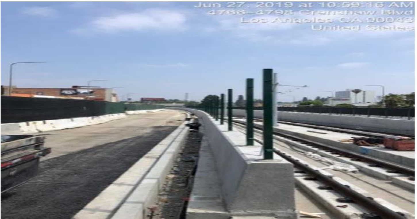
UG4- Installation of fence posts along southbound U-channel walls.
