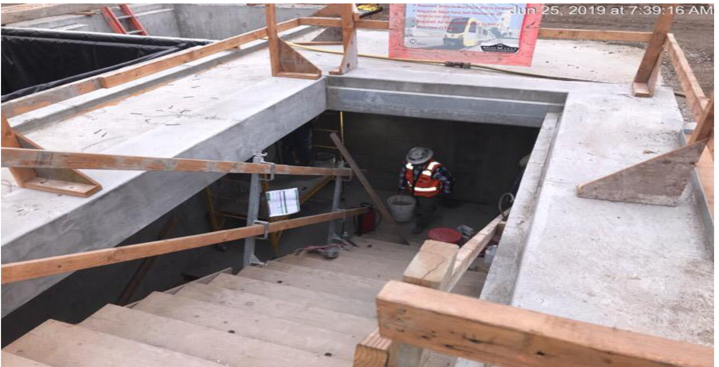
MARTIN LUTHER KING JR. STATION- Continued finish work from invert to concourse level at Emergency Exit #2.
