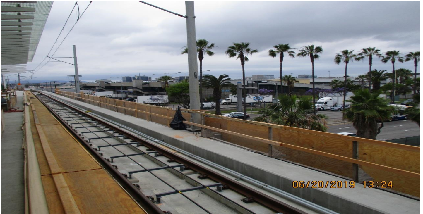
AVIATION/CENTURY- UP continue grout of North Bond track edge pavers and handrail at coping slab.
