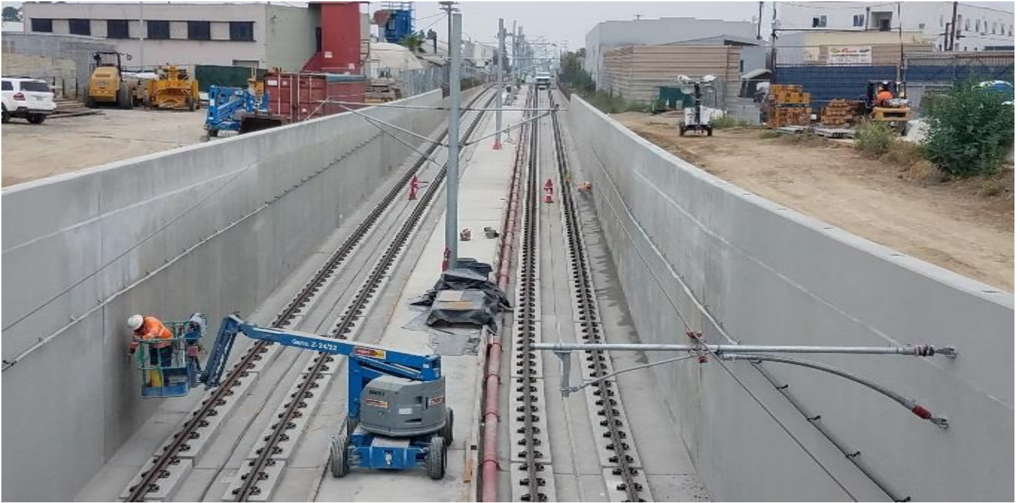
UG3- Continued finish work on U-channel walls of southbound portal.
