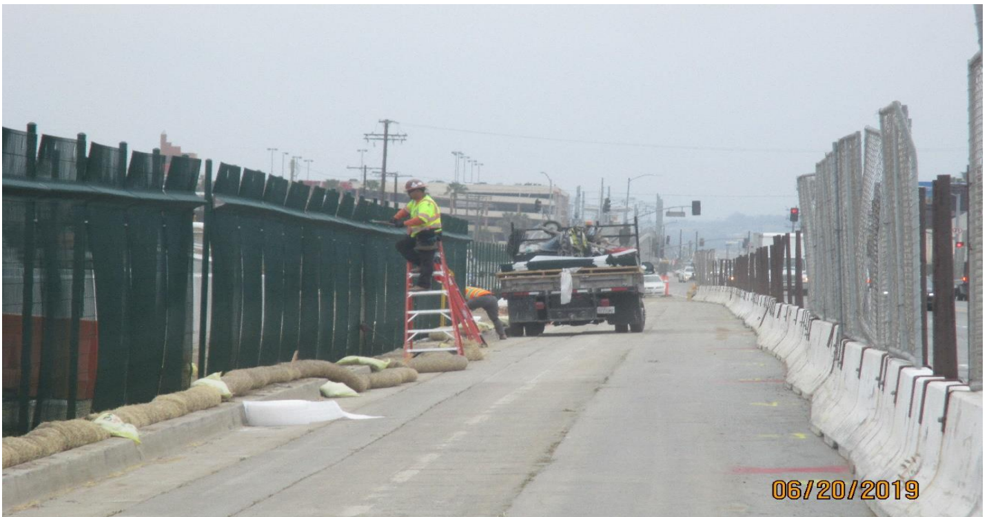
UG1- Erecting the wire mesh fence at UG-1.
