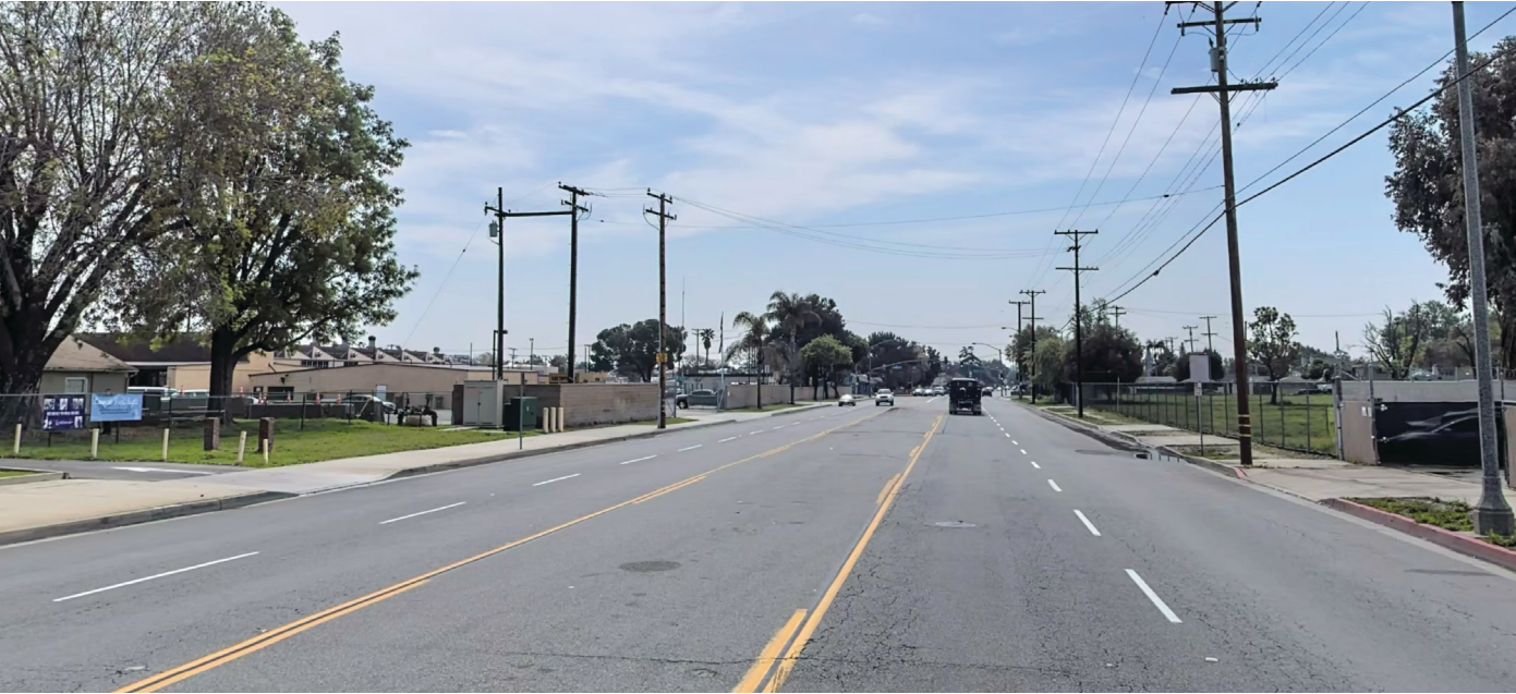
Garfield Ave Looking south towards Gardendale St.
