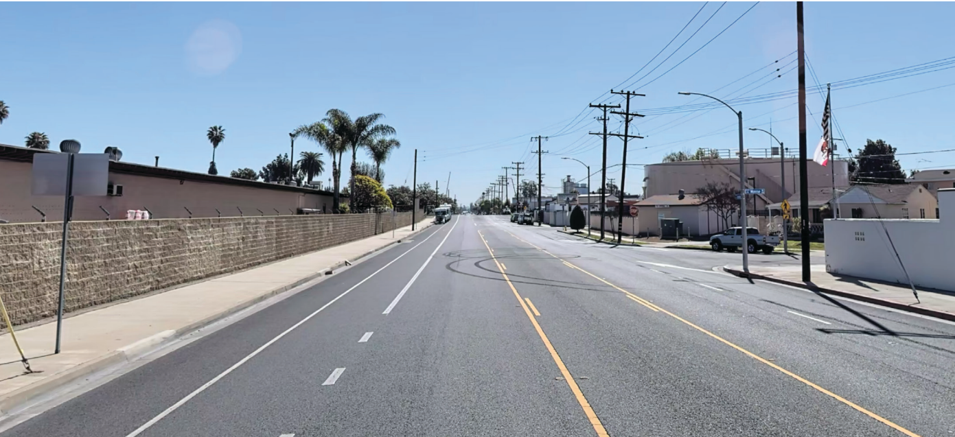
Gardendale St looking east towards ROW.
