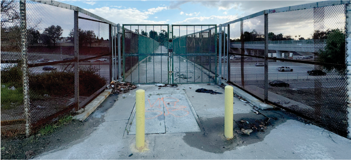
Arthur Ave Bridge, looking south towards I-105 Freeway
