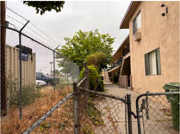
Eastern view of the southern boundary of the Subject Property
