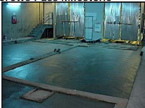
Above, Newly poured concrete glistens in the blue light of the "tail track" at the 7th/Metro station. Below, Wooden forms hold the wet concrete in place to form a plinth, or footing, for the reconstructed tracks. PHOTOS BY RODERICK PATES
