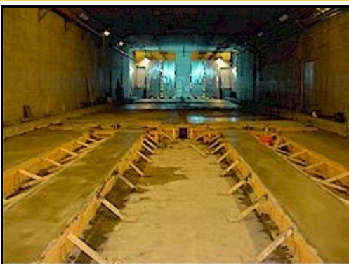
Above, Newly poured concrete glistens in the blue light of the "tail track" at the 7th/Metro station. Below, Wooden forms hold the wet concrete in place to form a plinth, or footing, for the reconstructed tracks. PHOTOS BY RODERICK PATES
