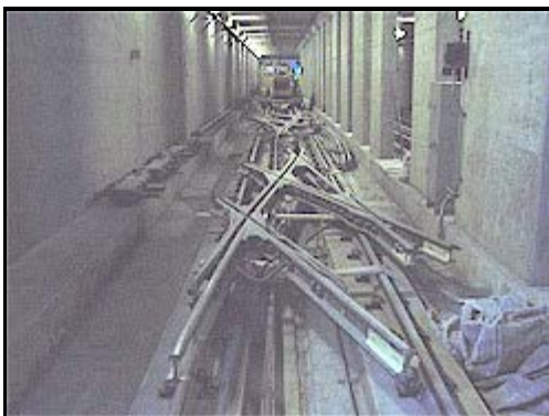
Above, large metal doors seal off the tail track construction area from the passenger platforms at the 7th/Metro station. Below, a double crossover, taken up earlier by construction crews, awaits installation on the new track bed. PHOTOS BY BILL HEARD
