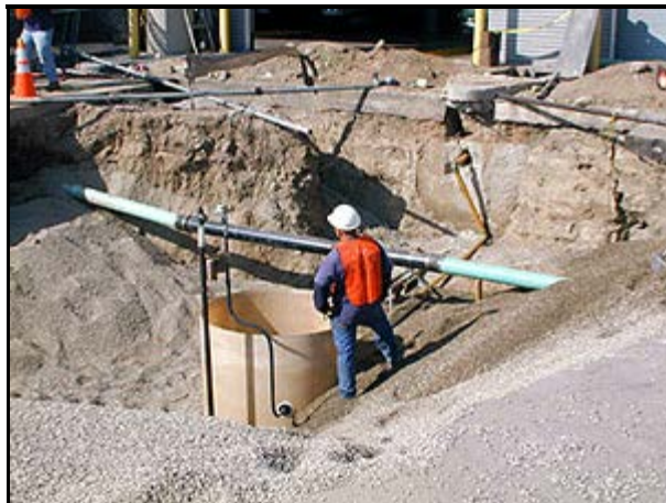
^ A worker stands next to the "collar" of an underground waste oil tank. Photo shows that retrofitting of the tank is almost complete.
