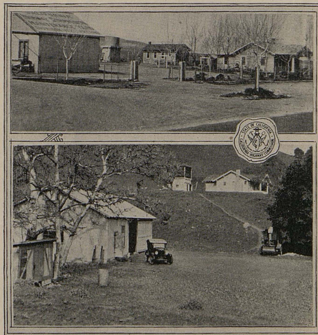
MAINTENANCE STATIONS—Above, a Division VI station on the trunk line in Kern County; below, home of a foreman on the Pacheco Pass Highway, Division IV.
