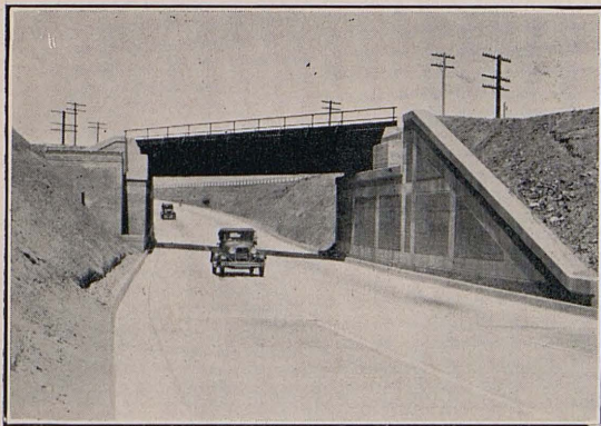
Subway at Califa in Merced County.
