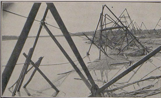
Tetrahedrons that saved the highway in the St. Francis flood.
