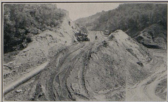
Grading operations on the Newhall alternate line.
