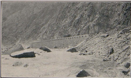
Slope paving and masonry walls.
