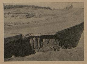
UNDERMINING of the old thin pavement at dip by flood waters. One hundred seventeen of these dips are to be replaced by culverts.
