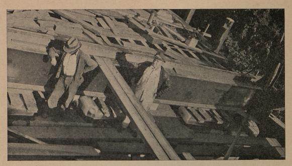
A MELTING SCENE—Here's the iceman helping the engineer watch six cakes of ice do the work of jacks in lowering bridge truss.
