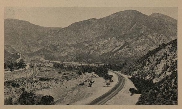
MINUS 59 CURVES, the Cajon Pass highway is shown after completion of the recent realignment operations. The channel of Cajon Creek has been changed, permitting a new route for the highway sufficiently removed from the hill slopes to prevent further blockades by the Blue Cut slide.
