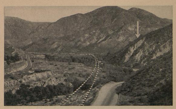
BEFORE MAJOR OPERATIONS by State engineers on the recently completed realignment project, the highway through Cajon Pass, famous transcontinental traffic gateway to southern California, had ninety-one curves, steep grades and the Blue Cut slide, indicated by arrow, that blocked the road with tons of dirt at every rain. One operation involved changing the creek channel to permit moving the road away from the slide.
