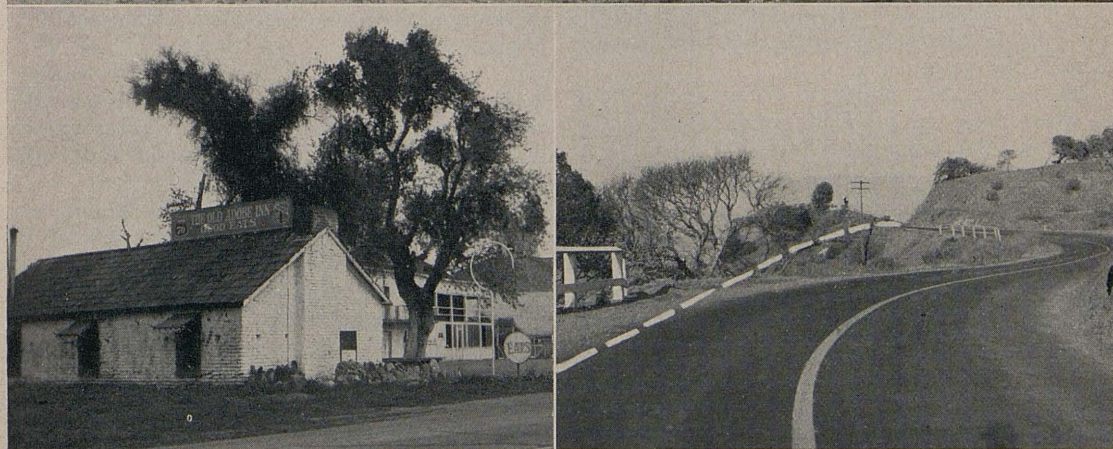
SOME 48 CURVES, mostly sharp ones, as shown in the top picture, distinguish the 3.3 miles of Pacheco Pass road from the summit easterly to the foot of the grade. New alignment indicated by dotted lines in the lower views will eliminate all short radius turns, widen the roadway and lessen grades. The historic San Luis adobe ranch house, 105 years old is shown at bottom.
