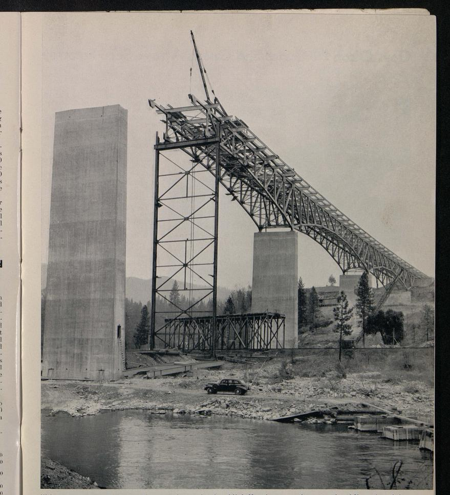
Highway bridge across Sacramento River at Antler on relocation of U. S. 99 made necessary by construction of Shasta dam. It is a steel deck truss structure 1330 feet long. The concrete deck will be 210 feet above the river
