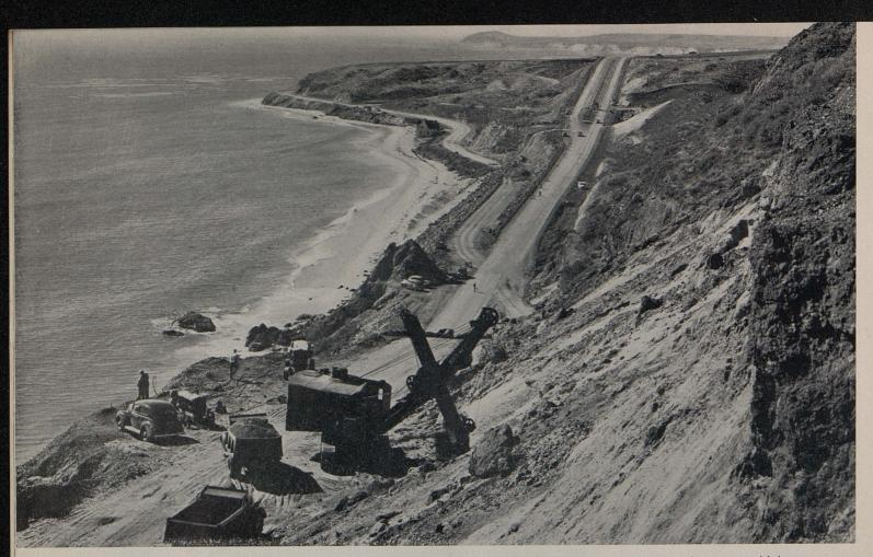
Two-yard power shovel removing 50,000 cubic yards deposit of beach sand on a bench 90 feet above coast highway
