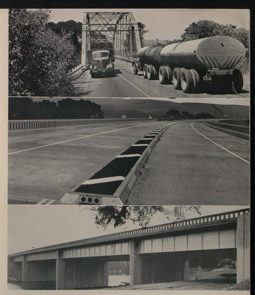
Upper—Antiquated bridge across Pajaro River at Sargent which has been replaced by new structure shown in lower photograph Center—Raised division strip on deck of new bridge contrasting with narrow roadway on old span
