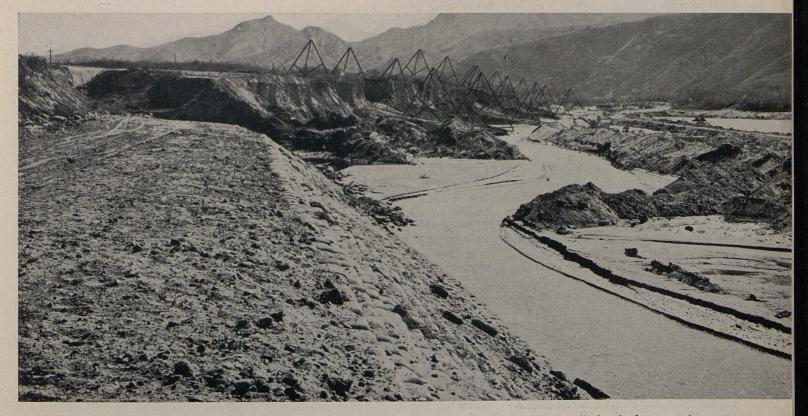
Thirty-foot steel rail tetrahedrons, shown in middle ground, and sacked concrete riprap installation in foreground
