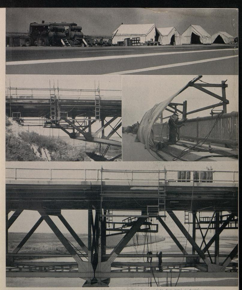
Top picture shows typical set-up of bridge painting equipment and camp. Center (left) painting superstructure from catwalks; (right) sandblaster at work on bridge railing. Canvas screen protects passing vehicles. Bottom—Raising catwalks on steel span over river
