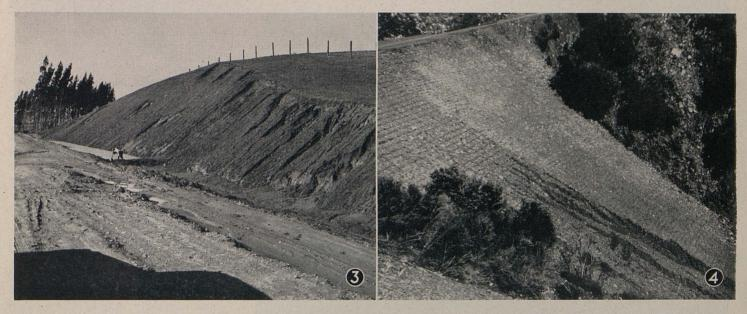
(3) Loss of top soil caused by first rain. No additional loss from subsequent rains has occurred. Soil is clay loam. (4) Fill slope protected by wattle method. On far half wattles were placed approximately 2 feet apart; on near half 4 feet apart. Note effects of erosion
