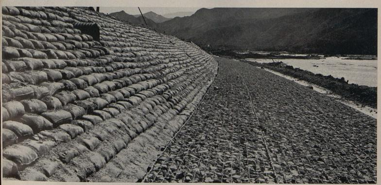
Sacked concrete riprap, 12 inches thick with rock and wire toe mattress, 8 inches thick and 14 feet 6 inches wide
