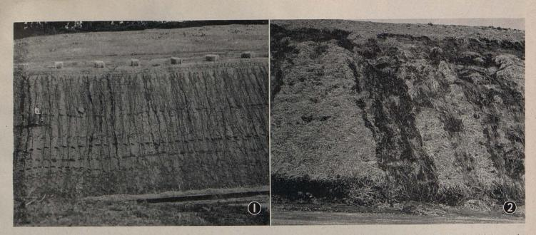
(1) Erosion gullies formed on a top soiled cut slope by 2.13 inches of rain. Note no intercepting drain ditches. (2) Result of 3 days rain, 3.95 inches in 24 hours, on newly treated slopes. Failure due to lack of bond of top soil to subsoil
