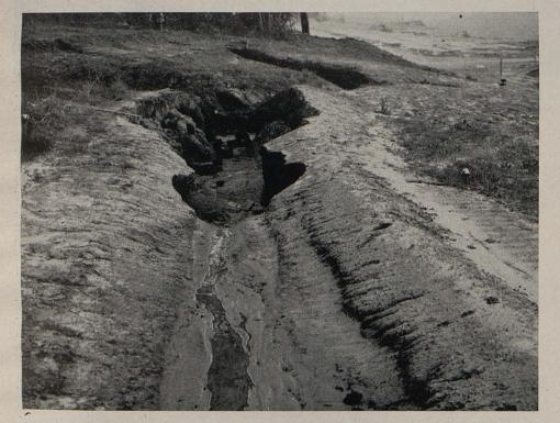
Intercepting drain ditches at top of slope like above also need vegetative protection
