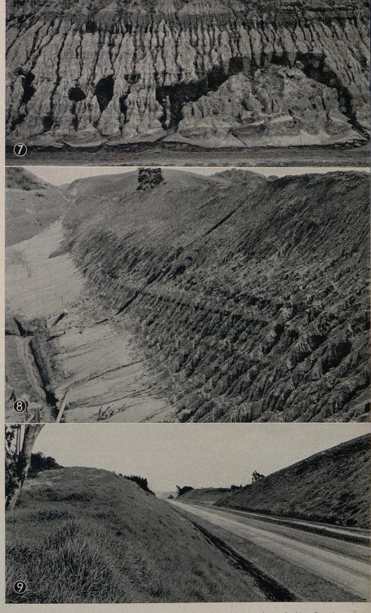
Typical erosion occurring on cut slopes during construction are shown in Nos. 7 and 8. On the same job and same soil 12:1 cut slopes are shown in No. 9 that were stabilized with top soil, rye grass and straw
