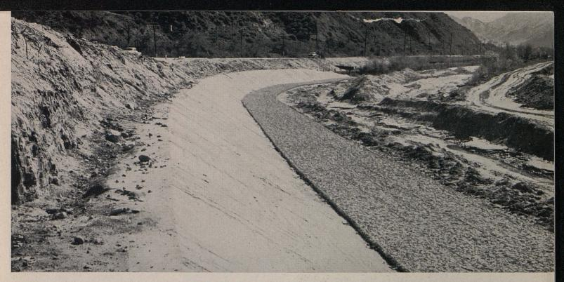
Portland cement concrete revetment on 11:1:1 slope 10 inches thick with rock and wire mattress 14 feet 6 inches wide
