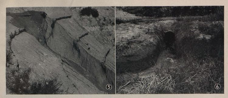
(5) Barriers that retard the flow of water are not successful. Note deep slip out. Highly erodible soils must not be allowed to move. (6) A down drain poorly installed. Water flows under pipe. Flattened and blanketed with humus material would promote grass growth over which water would flow without scouring
